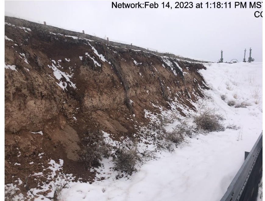
Photo # 9008 Slope stabilization BMP's insufficient.
