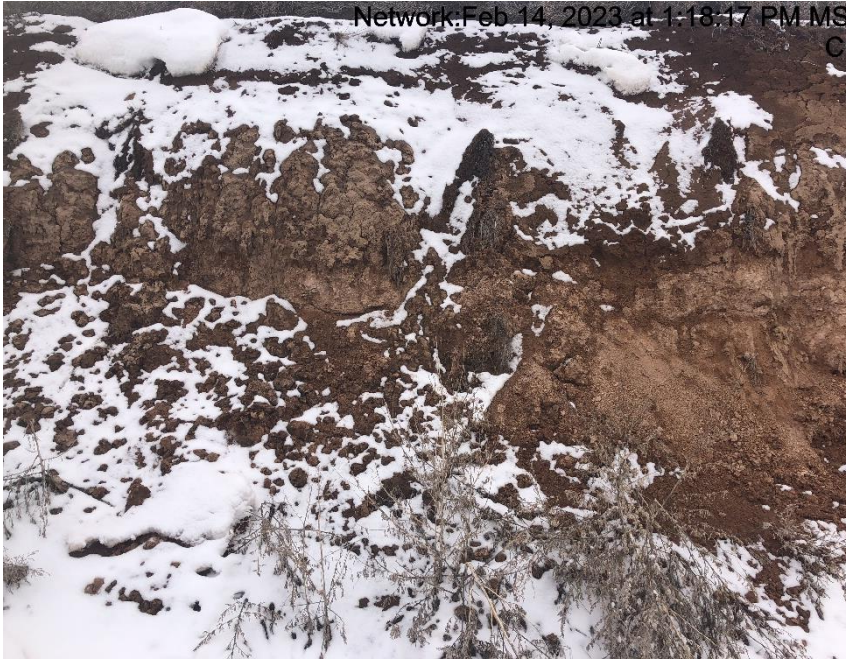
Photo #9009 Slope stabilization BMP's insufficient.
