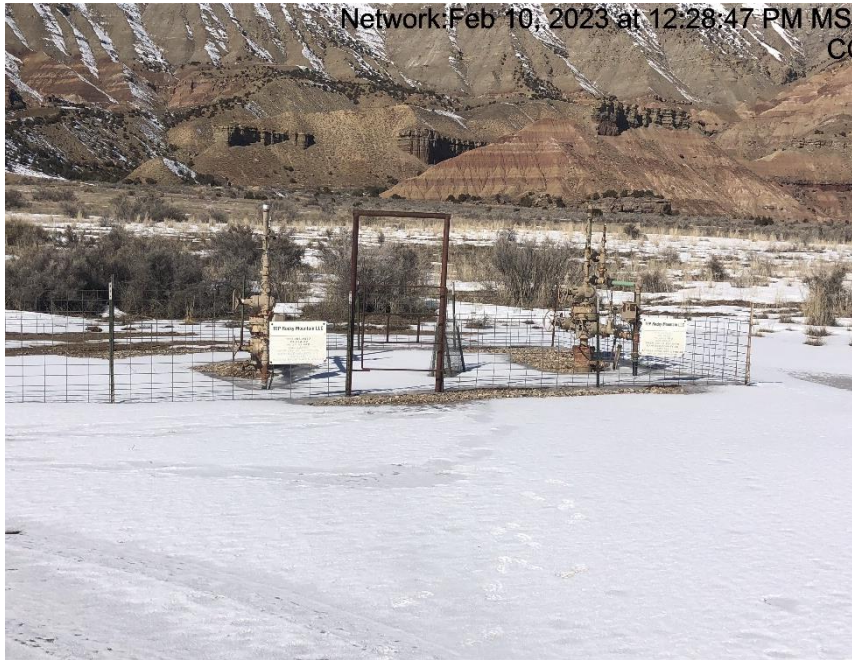
Photo #9001 Wellhead signs weathered and not legible.
