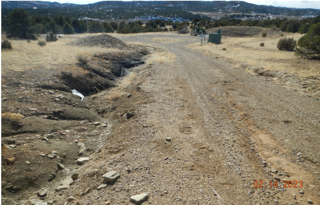
Photo 1. Facing southwest along the access road toward the location. The road side has eroded and needs to be repaired and stabilized.
