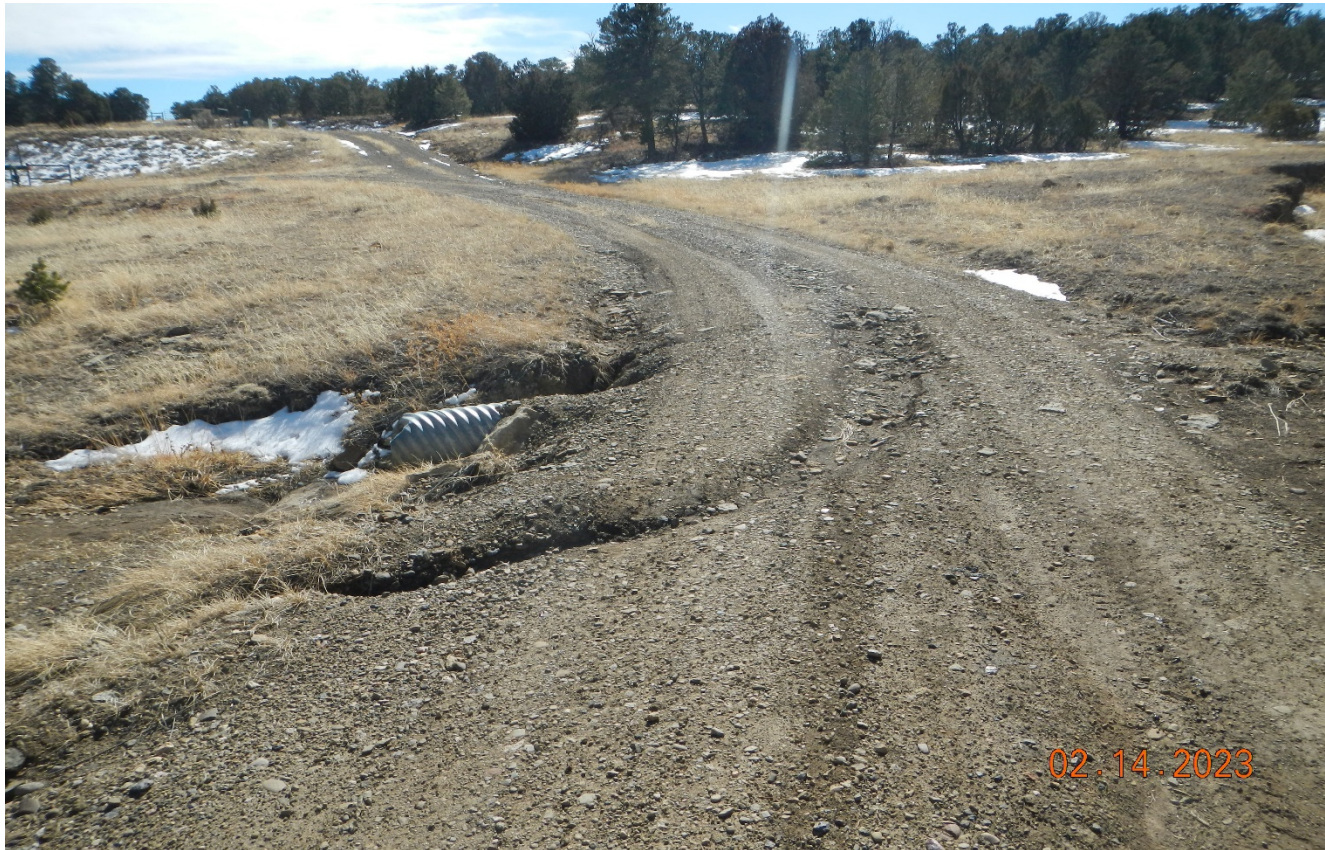
Photo 2. Facing south toward the access road. There is erosion at the culvert outlet that needs to be repaired. Corrective action not complete.
