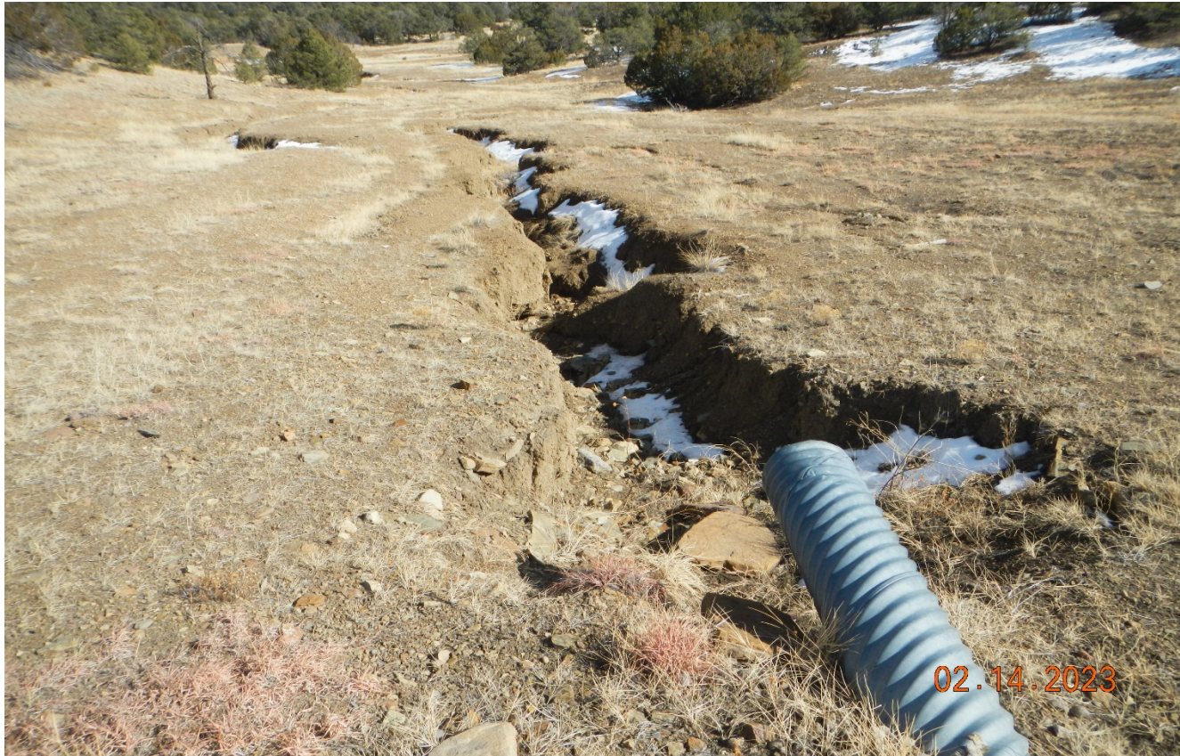
Photo 1. Along the main road at Lat/Long:37.14002,-104.68079. There is erosion at the culvert outlet that needs to be repaired. Corrective action not complete.
