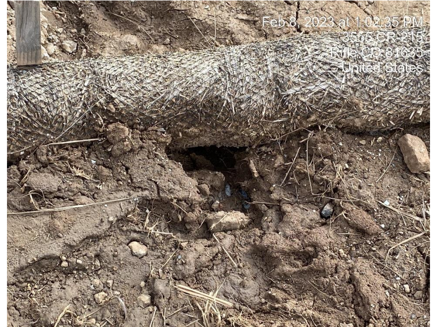
Erosion underneath wattle
