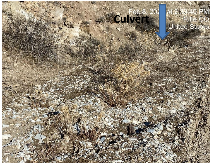
Plugged drainage ditch
