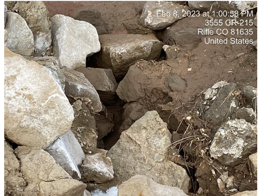
Sediment trap erosion
