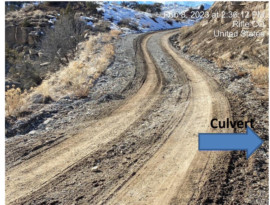
Plugged ditch diverting runoff over lease road
