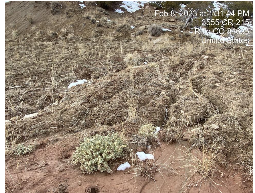
Soil erosion outside BMP
