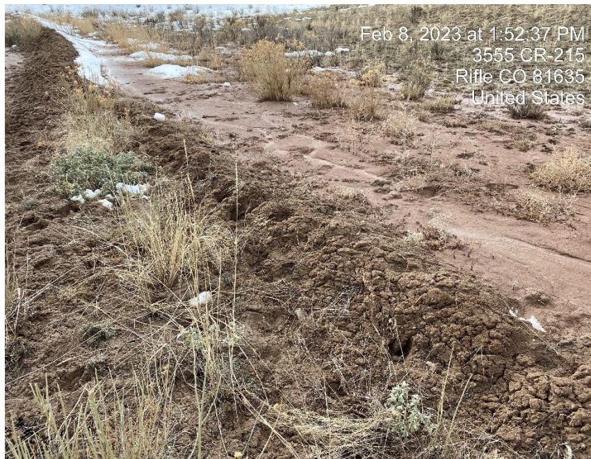
Sediment filled ditch
