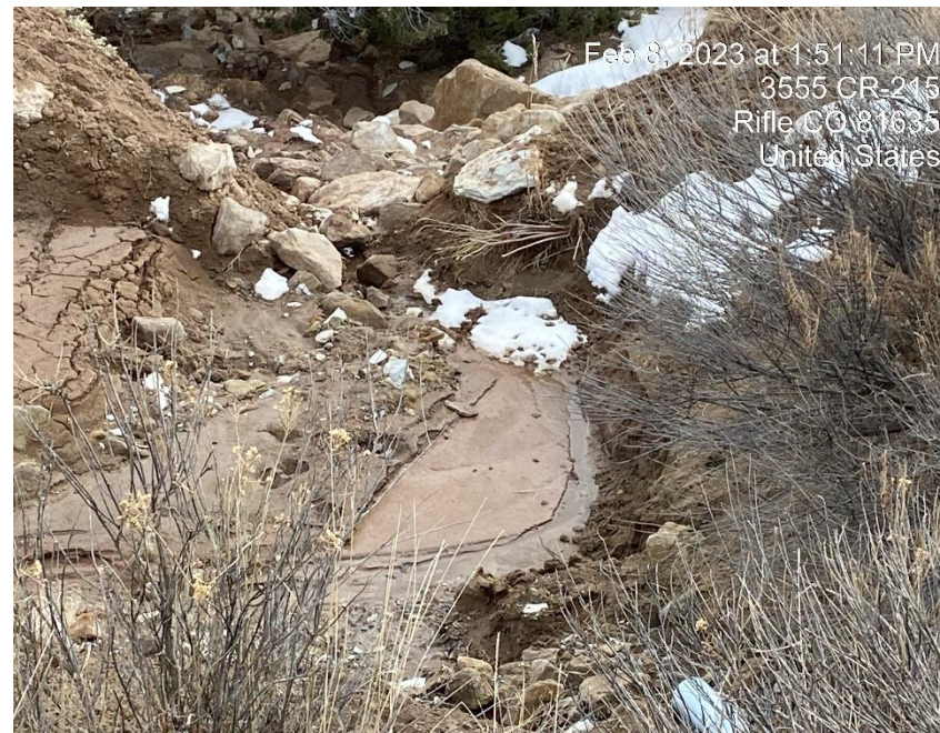
Washed out sediment trap
