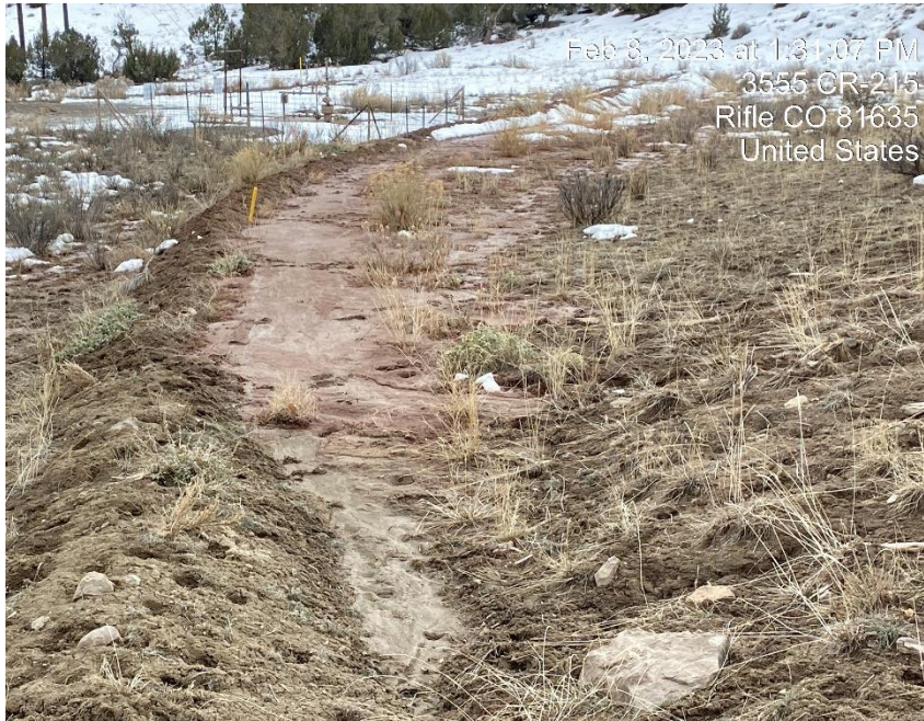
Sediment filled ditch
