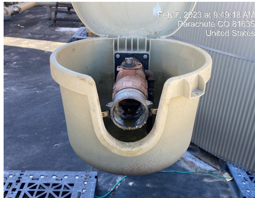
Uncapped loadline on produced water tank
