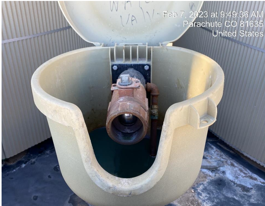
Open end loadline on condensate tank
