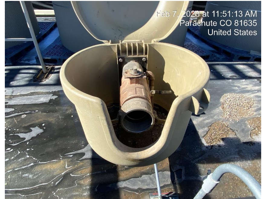
Open valve and open end loadline
