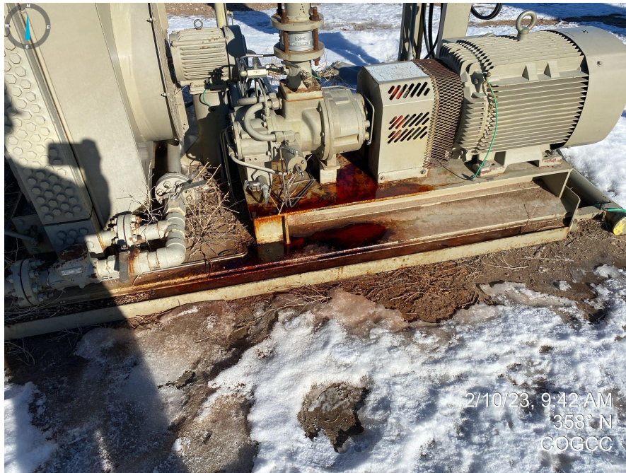
Photos 17 & 18. Unknown red fluid observed on skid of compressor, located on the northeastern portion of the location.
