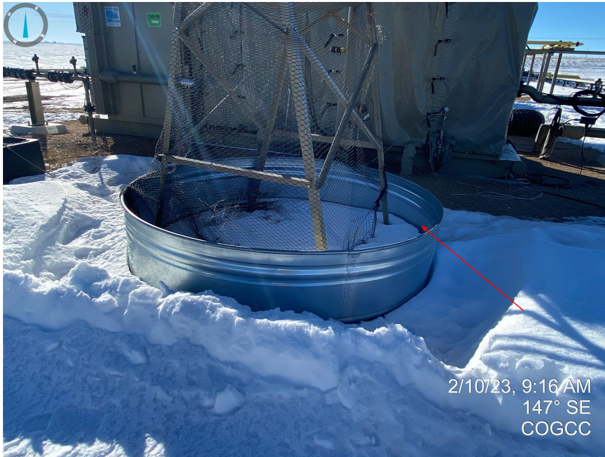
Photo 23. Facing southeast near the production equipment. Photo illustrates the the wildlife netting is inadequate and needs to be repaired to exclude wildlife entry to the secondary containment area.
