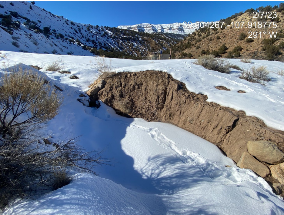
Photo 5. Photos show rill erosion occurring throughout BMPs to the southeast of the location, particularly on sediment trap walls. Trap erosion is acting as an additional sediment source.
