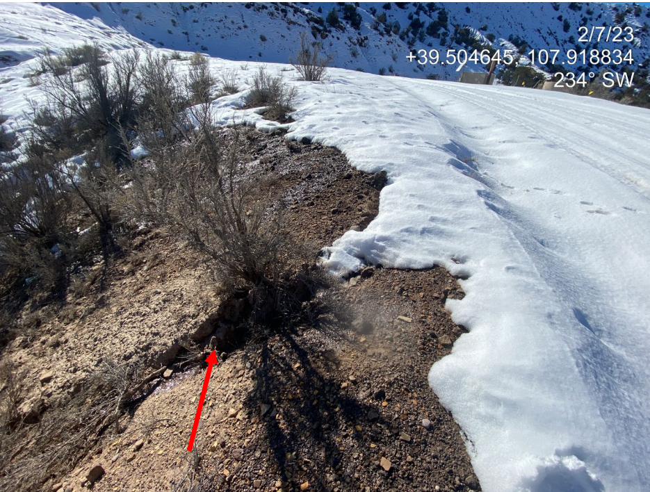
Photo 4. Photos show runoff from the access road causing erosion.
