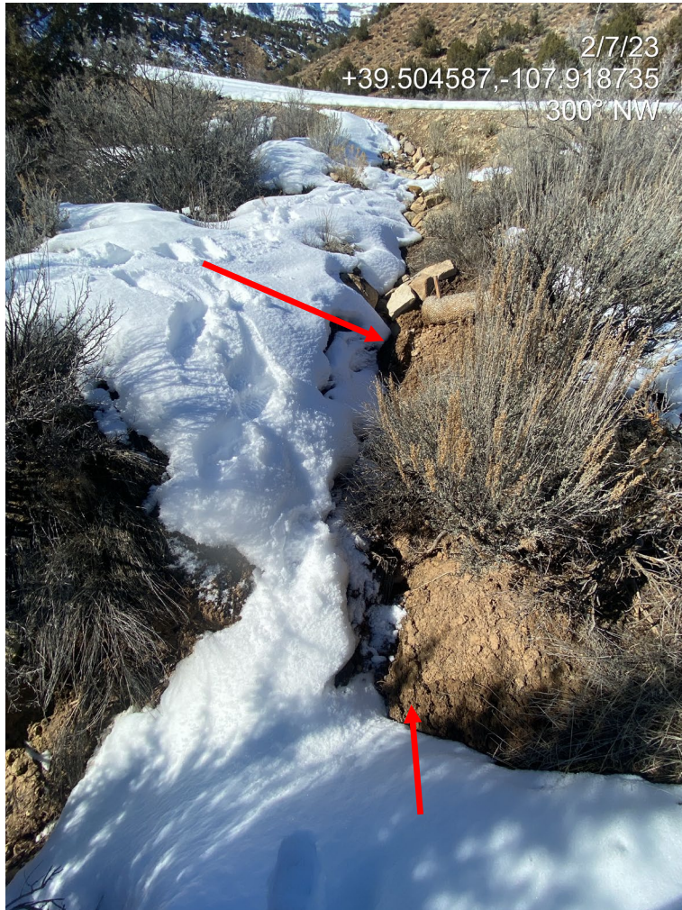
Photo 3. Photos show stormwater BMPs to the south of the access road. Stormwater discharged from the BMPs is causing scouring resulting in gully erosion (right).
