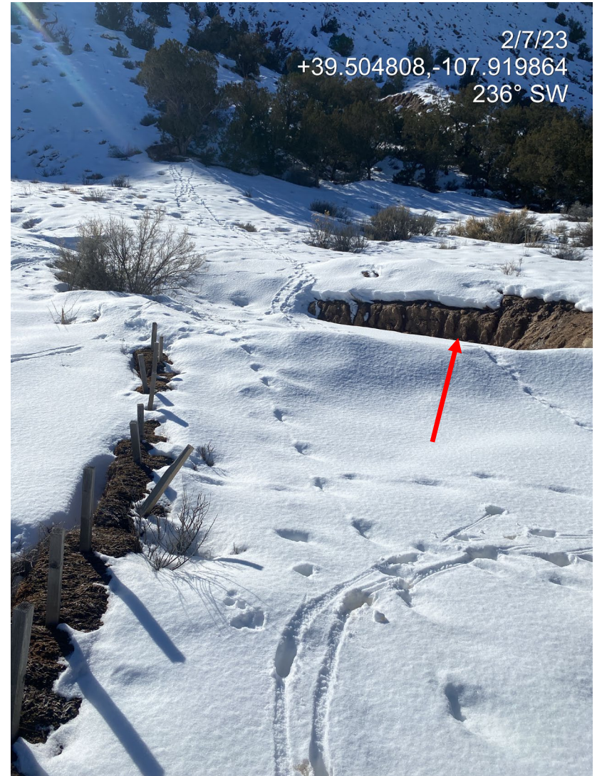
Photo 8. Photos shows additional BMPs which are snow covered. Follow up inspection required to assess snow covered areas. Note erosion degradation in sediment trap to the northwest (right).
