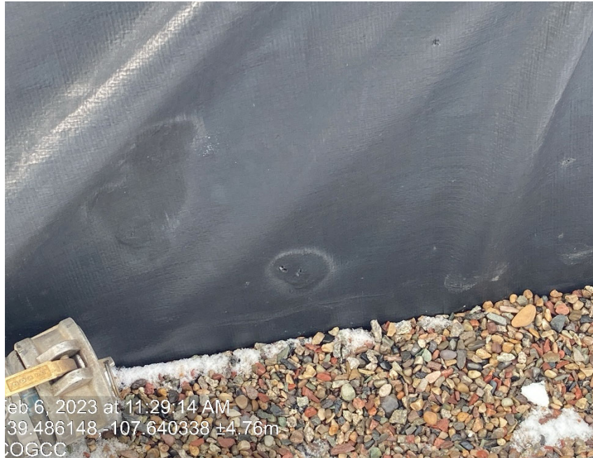
Holes in containment
