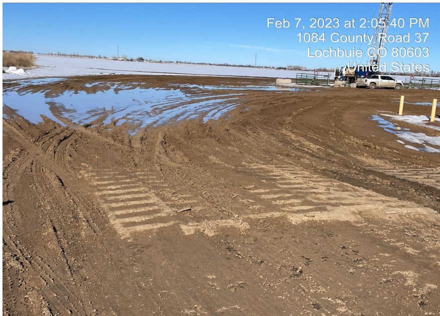
Photo 4. Entrance of location looking north of vehicle tracking device BMP is in non-proper functioning condition.
