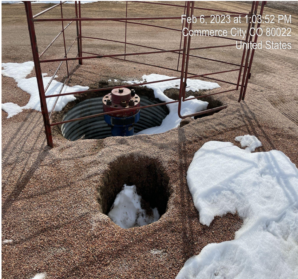
Photo 5. Photo taken on location next to well Alma west 26W-20-03. Large hole outside of fenced area no protective barrier to humans or wildlife present.
