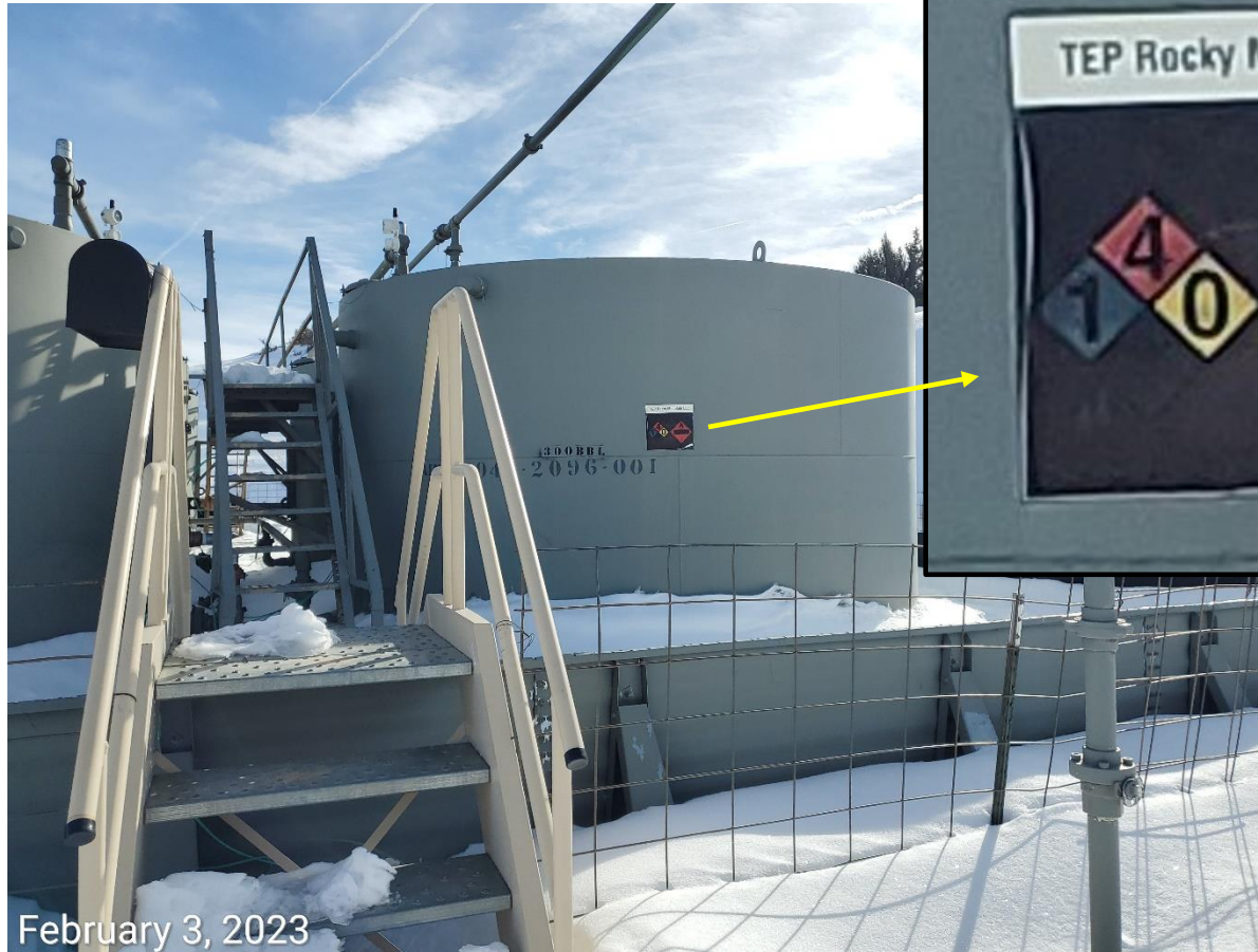
Photo 3: Photo shows labeling on tank is no longer legible.
