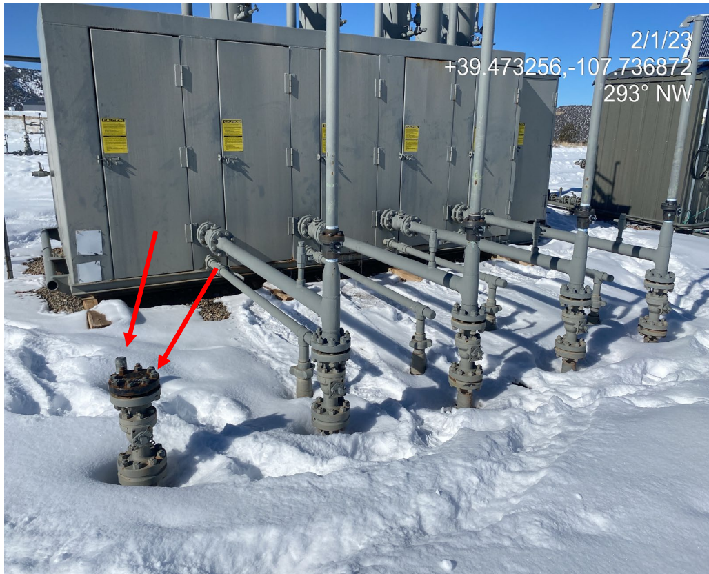
Photo 2. Photos show two (2) risers which appear to be associated with a plugged and abandoned well and decommissioned flowline.
