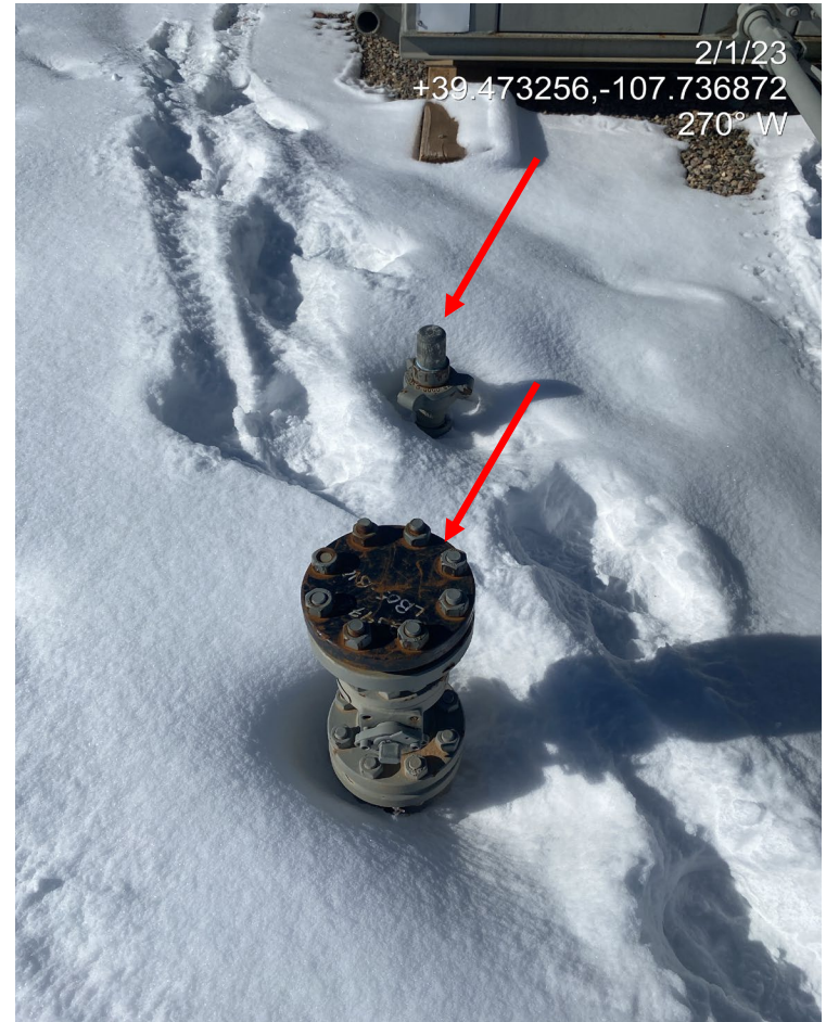
Photo 2. Photos show two (2) risers which appear to be associated with a plugged and abandoned well and decommissioned flowline.
