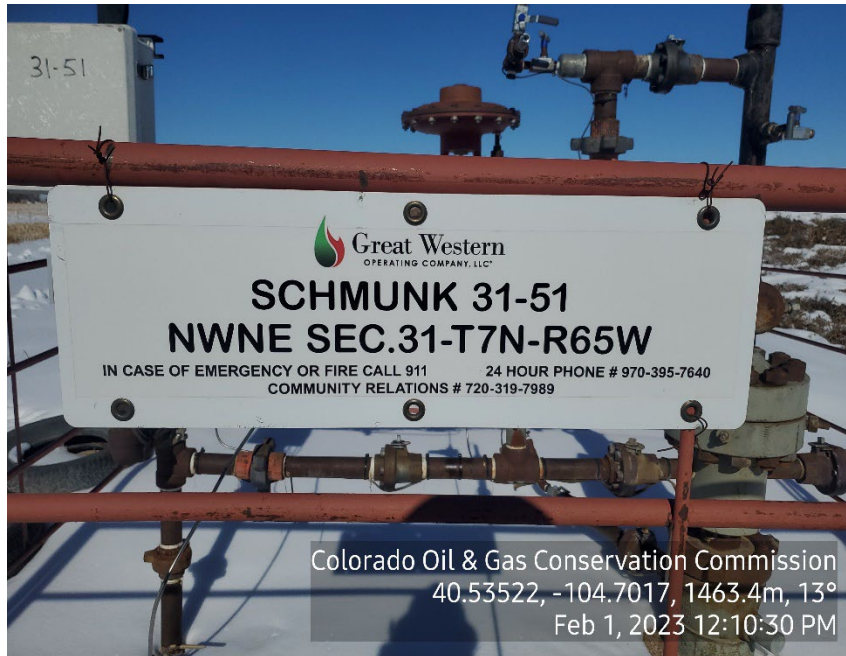
Photo 1: Wellhead Sign; INCORRECT OPERATOR/EMERGENCY #
