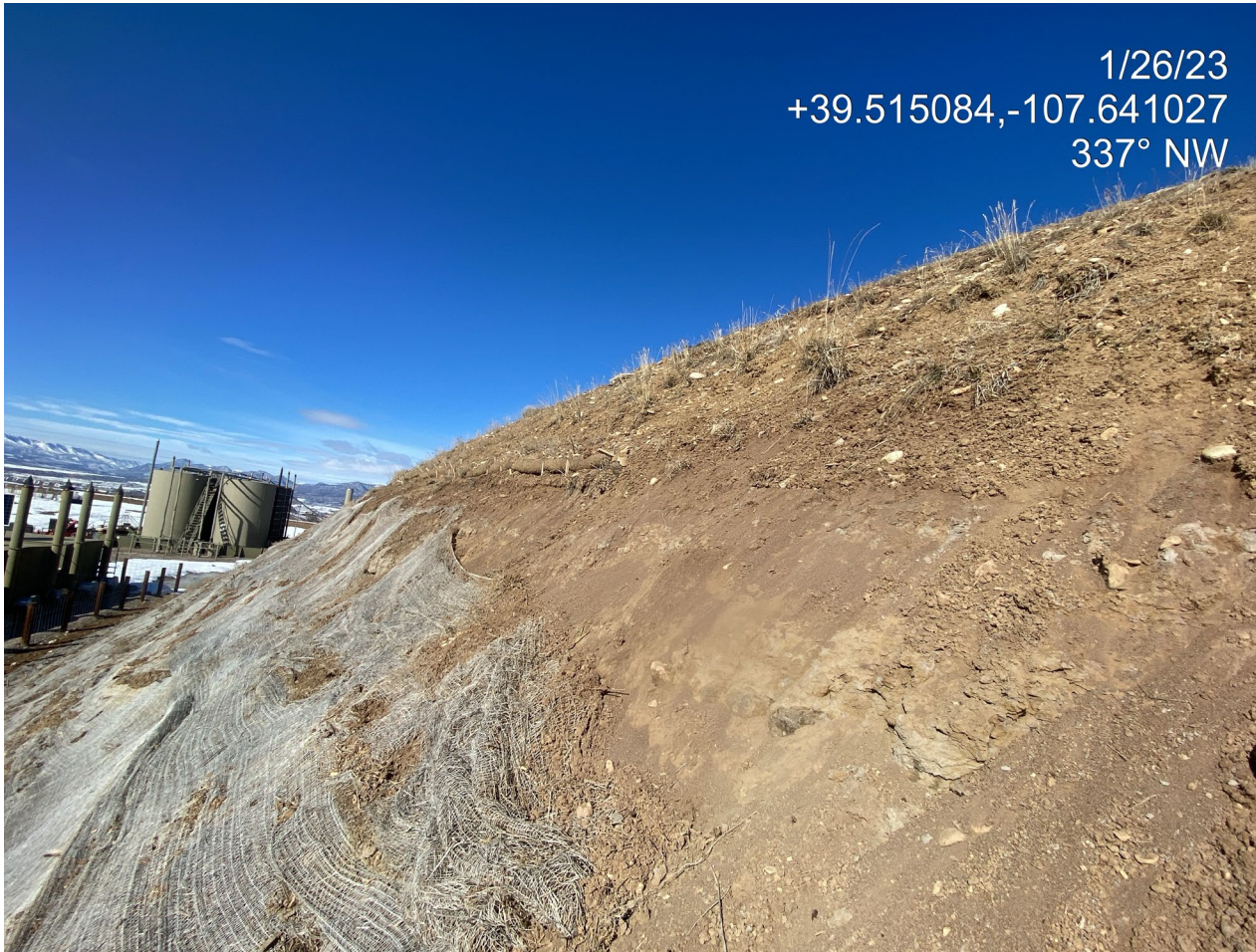
Photo 5. Photo shows BMP degradation and cut slope erosion. Soils were observed to be actively falling from the slope from gravity (not wind or water) indicating a particularly unstable slope. See also attached video.
