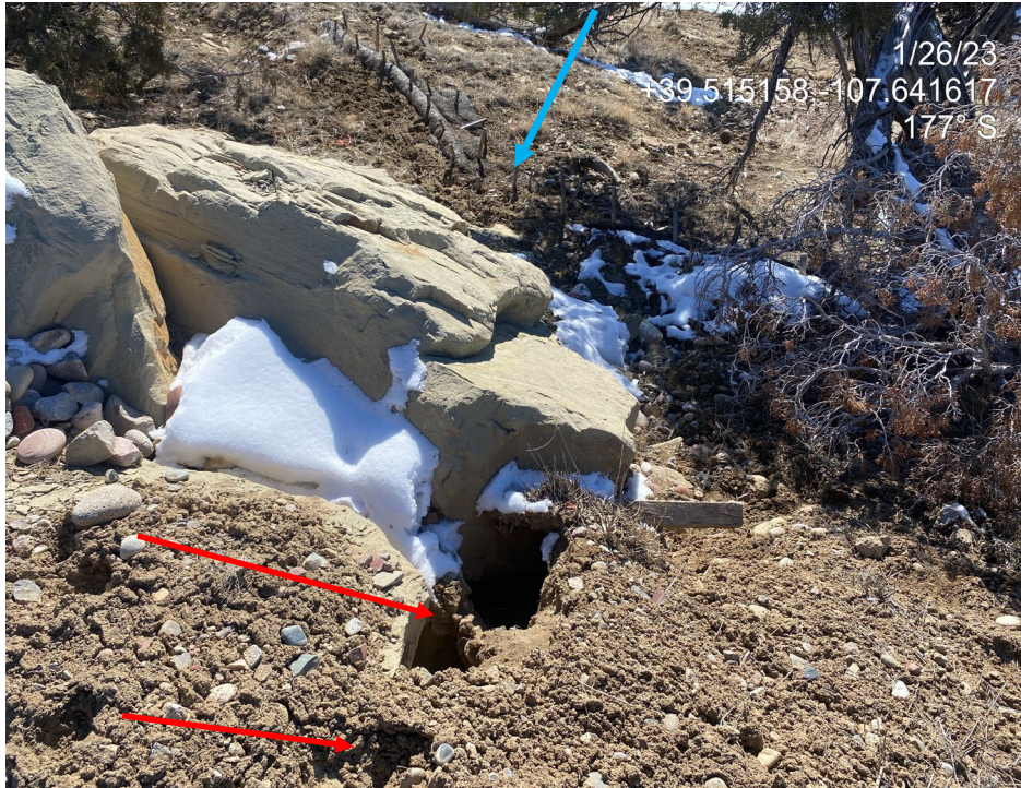
Photo 7. Photos taken from the southern edge of the location shows where stormwater is undermining/cutting beneath rip-rap, armoring the fill slope (left, red arrow). A wattle installed below has been overtopped (blue arrow, right).
