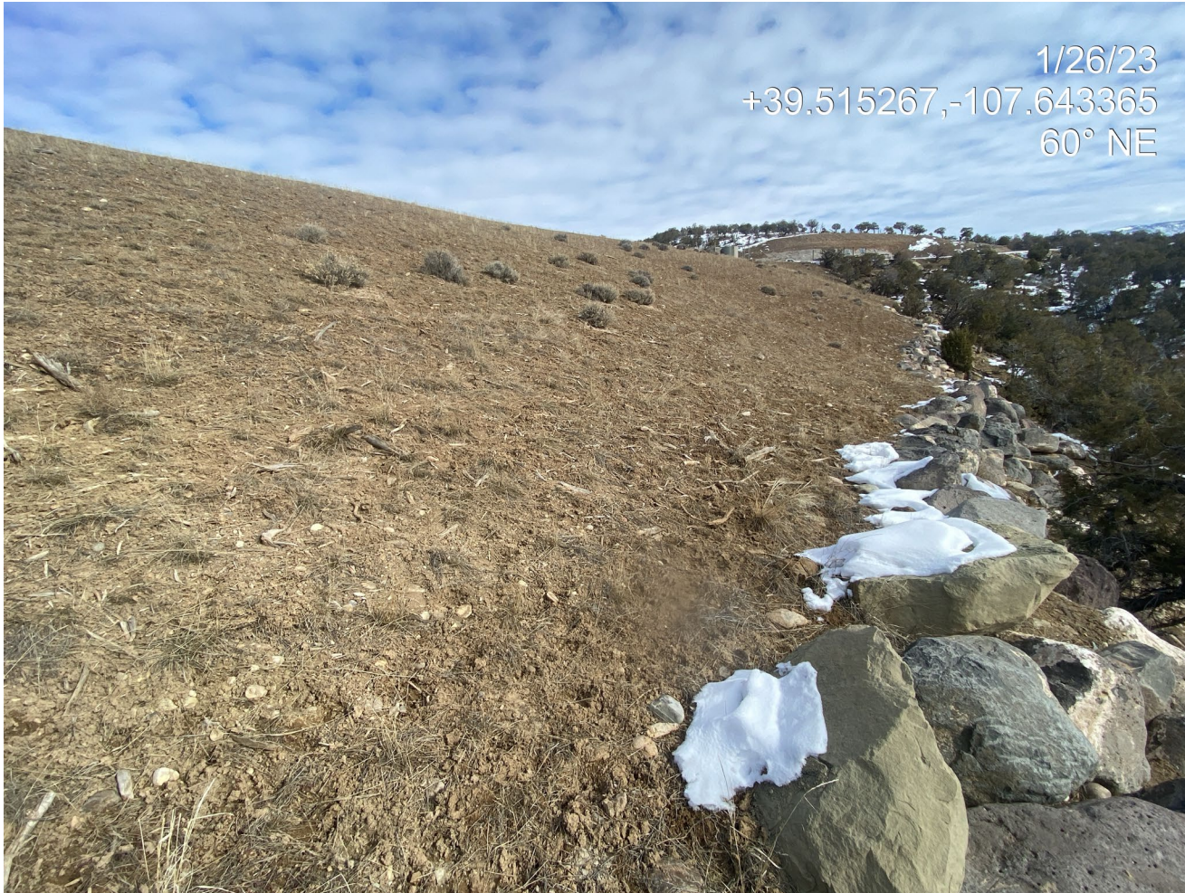
Photo 11. Photo shows the interim area/fill slope at the southwest of the location. The slope appears sparsely vegetated with perennial grasses.
