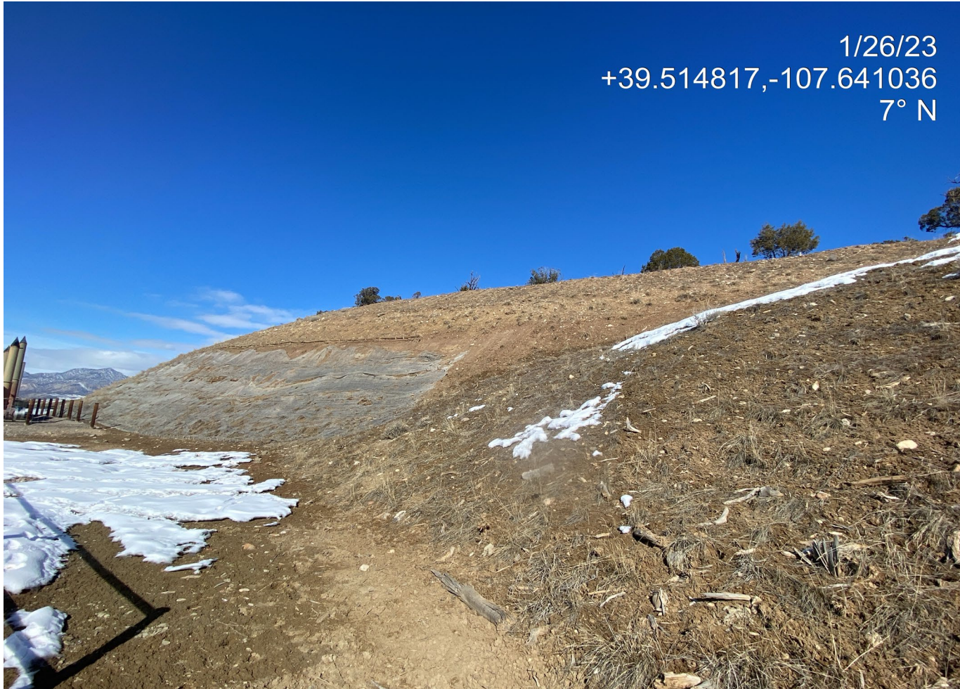
Photo 3. Photo taken at the east of the location shows an overview of the eroding cut slope behind the separators.
