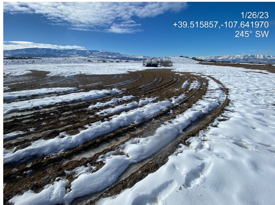
Photo 2. Photos show degradation to the pad surface and a lack of stabilization BMPs and tracking controls.
