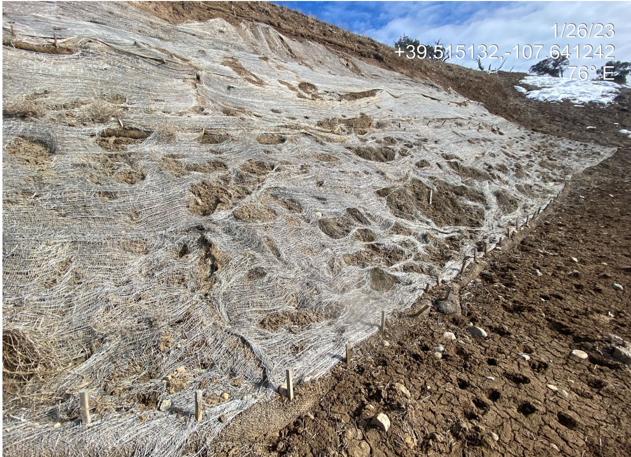
Photo 4. Photos taken at the east of the location show the cut slope behind the separators. The erosion blanket is degraded, sediment has overtopped wattles, stabilizing perennial plants appear sparse. Sediment is accumulating at the base of the slope.
