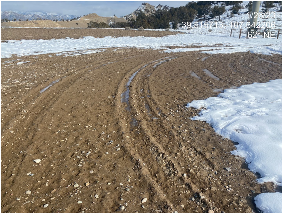
Photo 2. Photos show degradation to the pad surface and a lack of stabilization BMPs and tracking controls.
