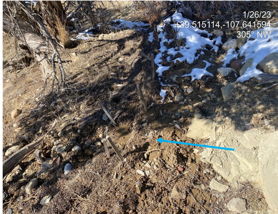
Photo 7. Photos taken from the southern edge of the location shows where stormwater is undermining/cutting beneath rip-rap, armoring the fill slope (left, red arrow). A wattle installed below has been overtopped (blue arrow, right).
