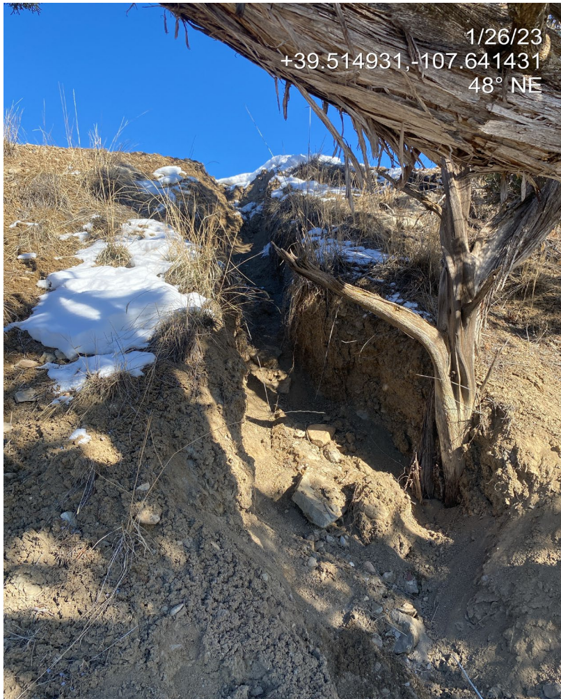
Photo 6. Photos taken to the south of the separators, where the working pad meets the access road shows a large gully.
