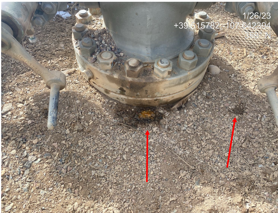
Photo 8. Photos show staining at wellheads.
