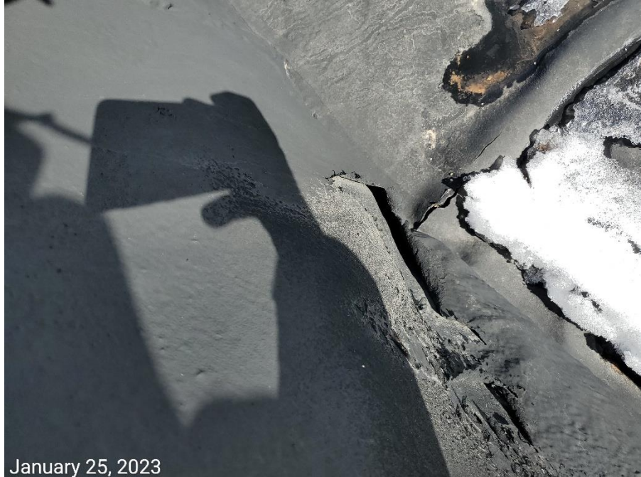
Photo 3: Tears/rip apparent at base of the liner. Liner does not appear to be impervious.
