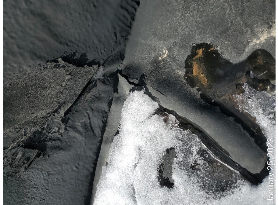
Photo 3: Tears/rip apparent at base of the liner. Liner does not appear to be impervious.
