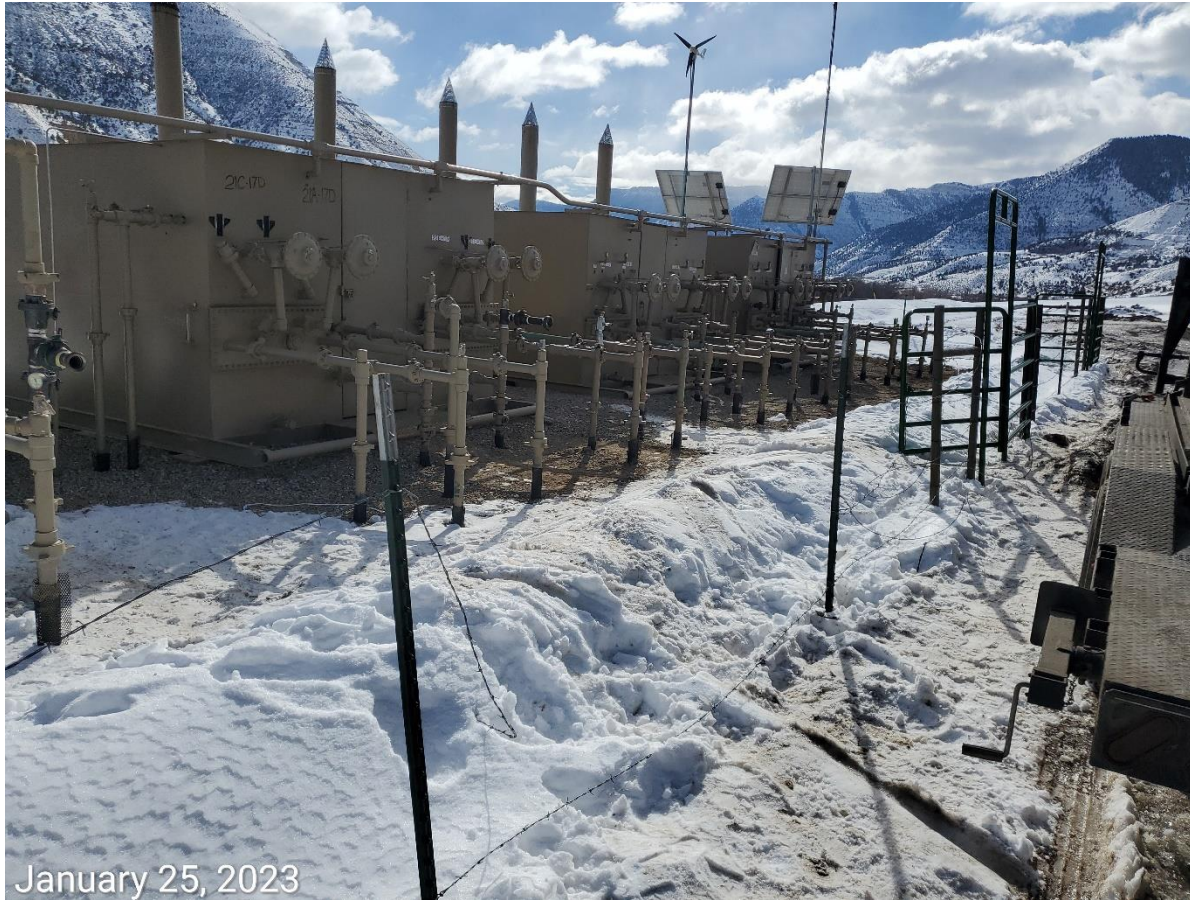
Photo 3: Fence in disrepair at the separator equipment.
