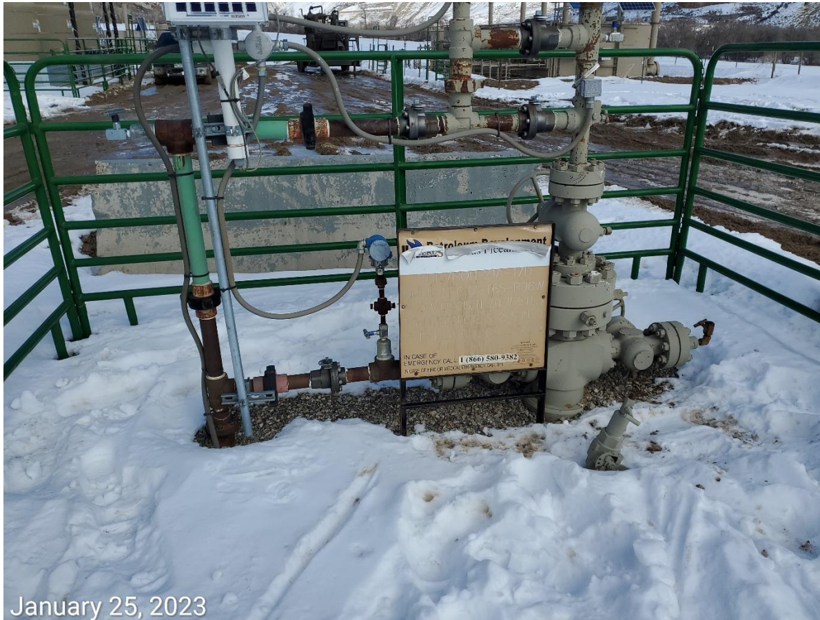
Photo 4: Photo example showing Operator information label applied to the wells is peeling. Maintenance advised to ensure signage remains legible.
