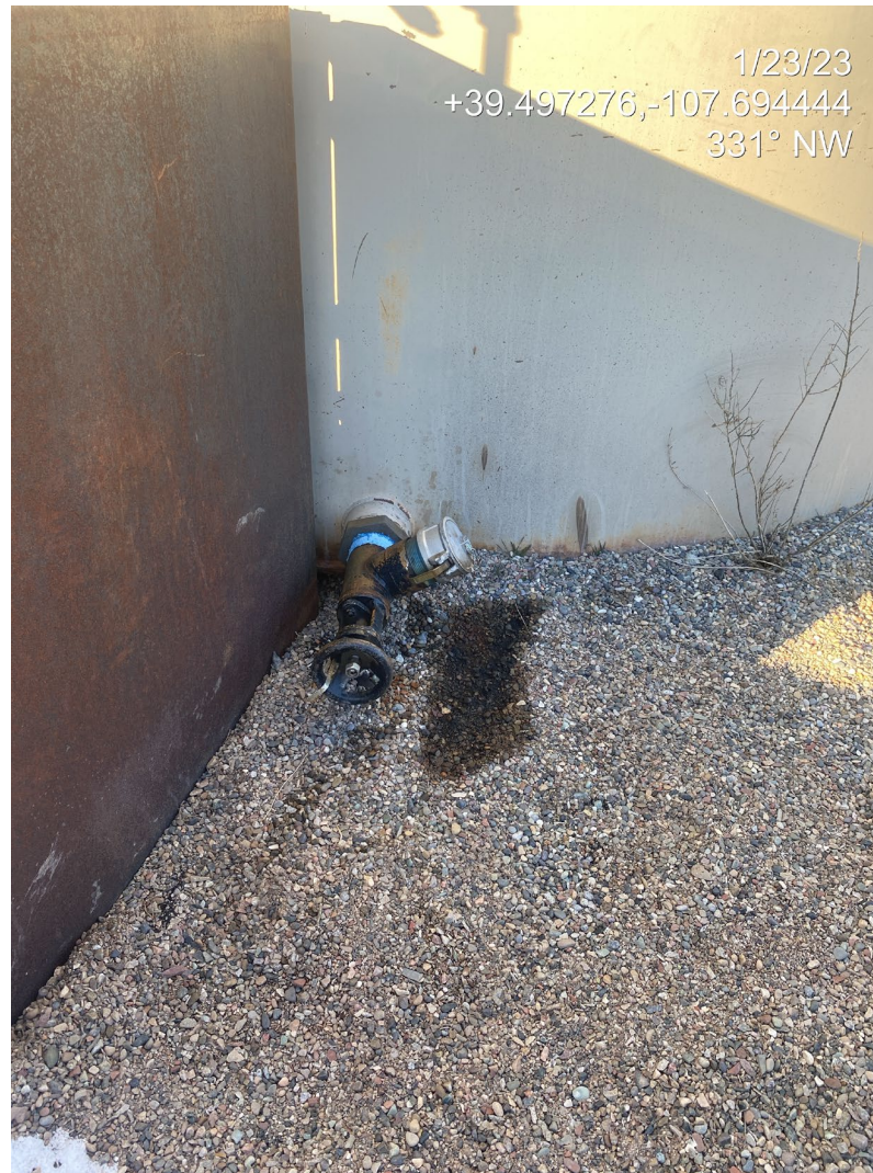
Photo 4. Photo shows staining beneath a produced water tank drain line.
