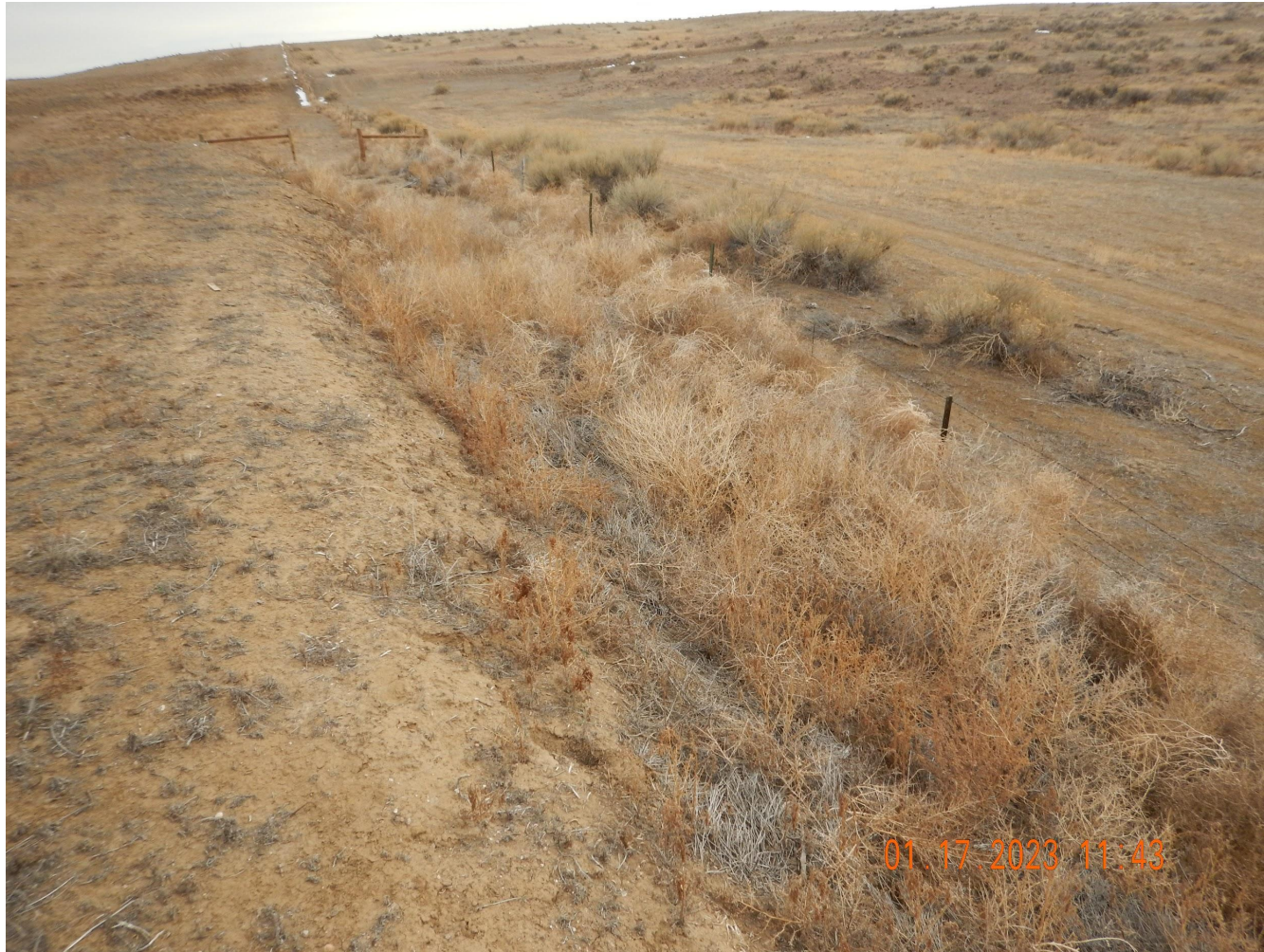
Photo 7. Photo taken from the southeastern location, facing East. Photo illustrates weedy vegetation along the fenceline which is considered weed debris and needs to be removed.
