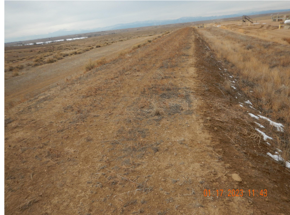
Photo 6. Photo taken from the southeastern location, facing West. Photo illustrates vehicle traffic on the topsoil stockpile which is in violation of Rule 1002.c.
