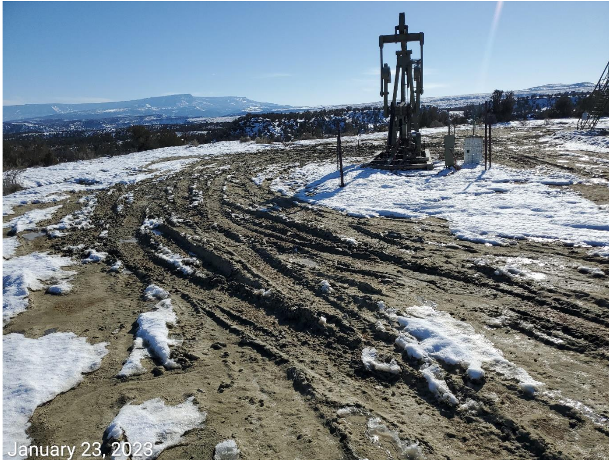
Photo 2: Photos example showing BMPs to stabilize the Location, and to minimize tracking and sediment transport remains missing or insufficient.
