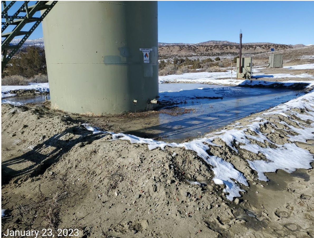
Photo 8: Photo taken from the tank battery. Vegetation remains evident within the secondary containment; secondary containment is not in proper functioning condition, or adequate in size to contain a spill from the tank. Vegetation within BMP compromises the impermeability of the containment.
