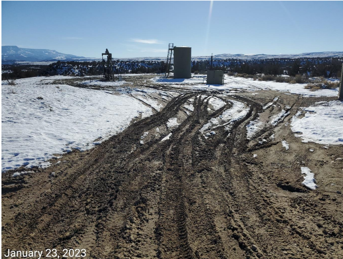
Photo 1: Photo taken from the Location entrance facing south. Photos example showing BMPs to stabilize the Location, and to minimize tracking and sediment transport remains missing or insufficient.
