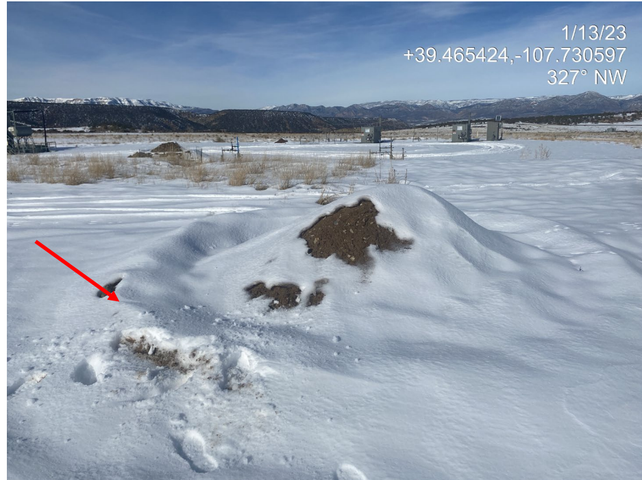
Photo 3. Photos show soil stockpiles from the plugged and abandoned well (left) and flowline (right) excavations. Excavated soil is surrounded by a berm of loose, unconsolidated soil.
