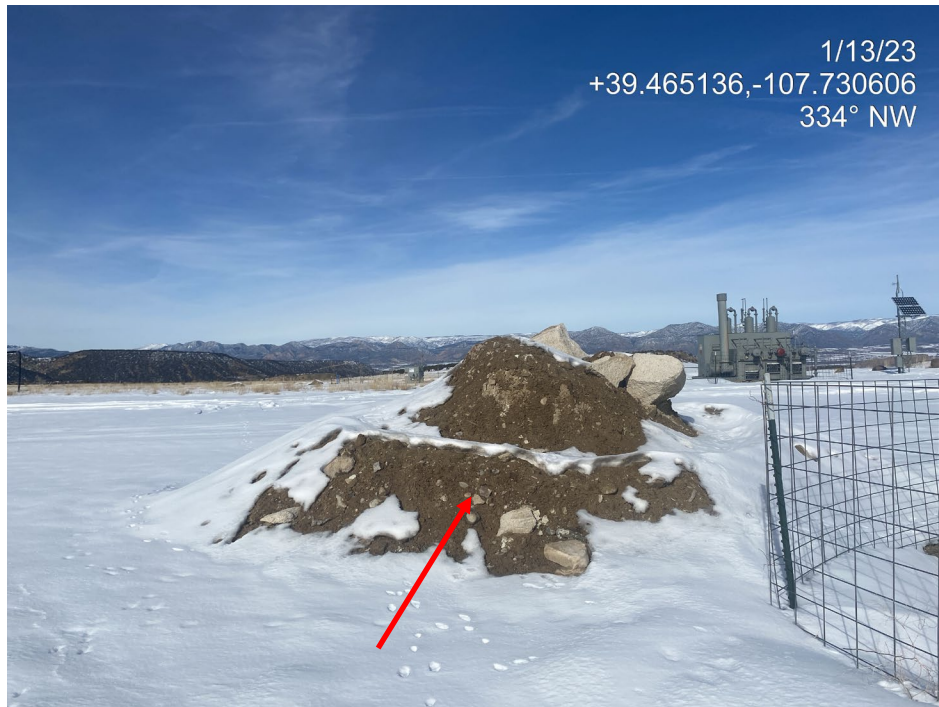
Photo 3. Photos show soil stockpiles from the plugged and abandoned well (left) and flowline (right) excavations. Excavated soil is surrounded by a berm of loose, unconsolidated soil.
