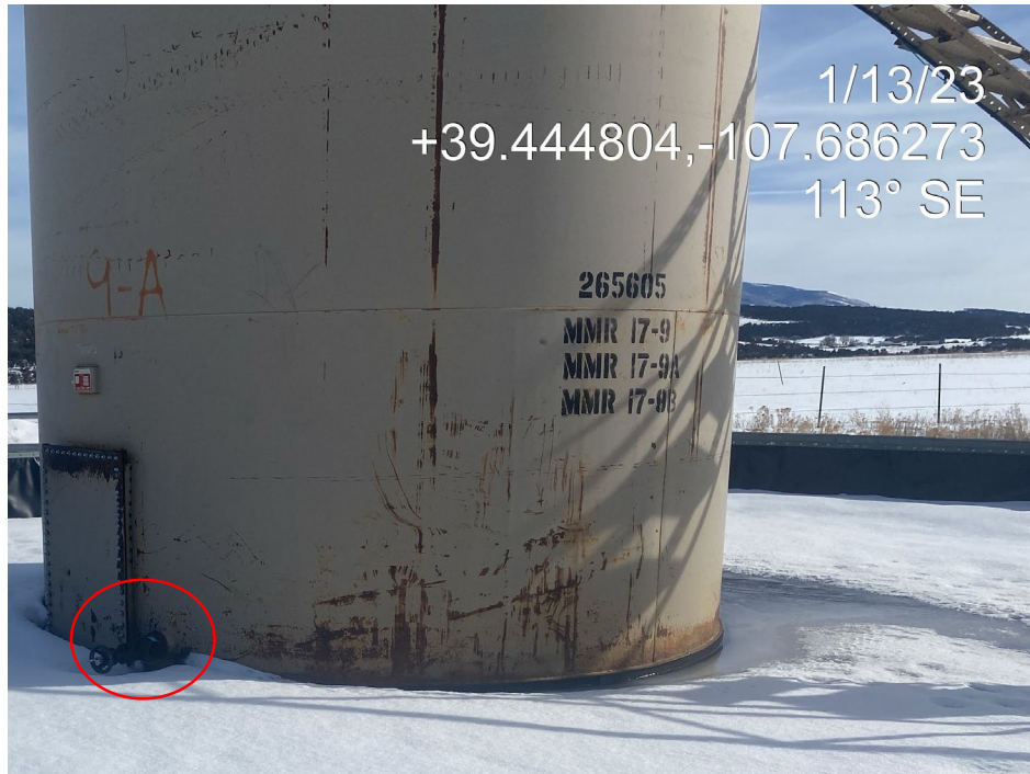
Photo 3. Photos shows a bull plug not installed on the tank drain (left) and wildlife protection BMPs are absent on the produced water secondary containment tank (right).
