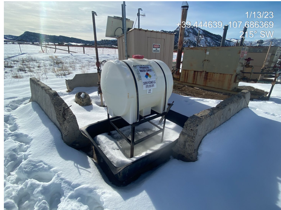
Photo 3. Photos shows a bull plug not installed on the tank drain (left) and wildlife protection BMPs are absent on the produced water secondary containment tank (right).
