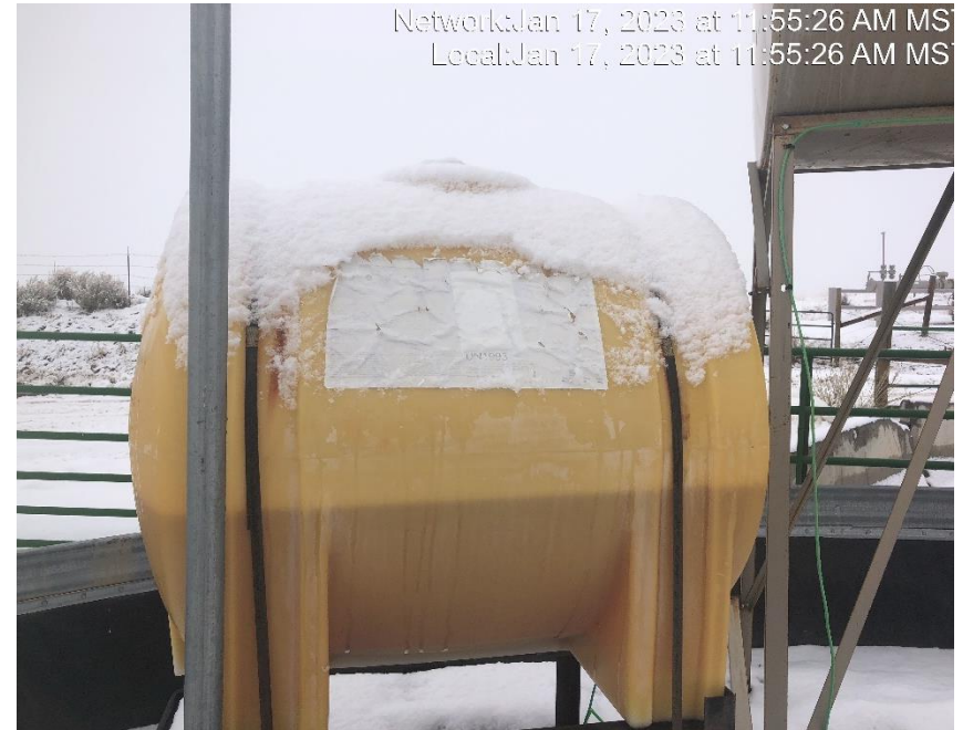
Photo #8789 Chemical tank label weathered and not legible.
