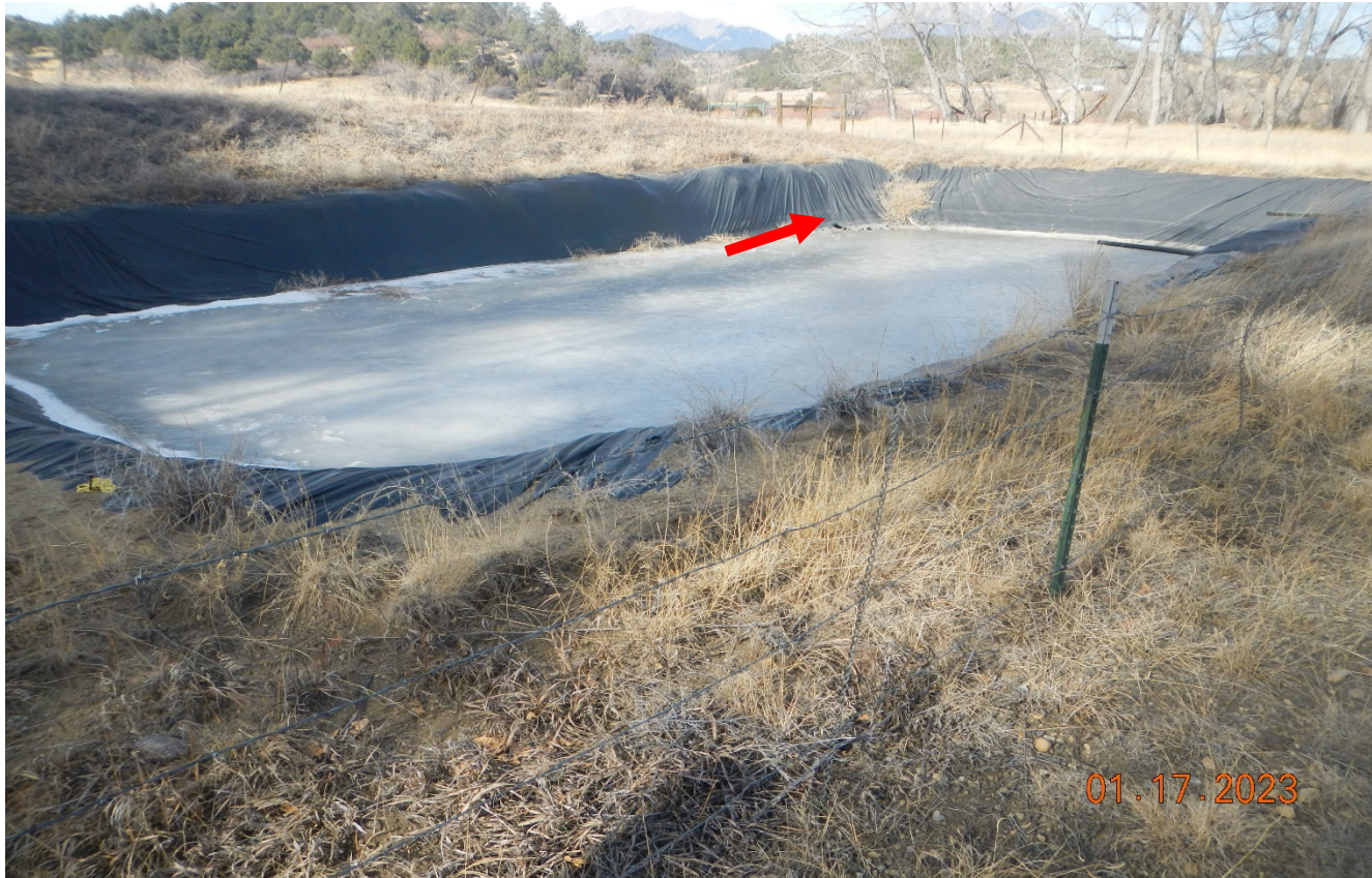
Photo 2. There are holes in the pit liner which need to be replaced. The water level at the pit has not been lowered.
