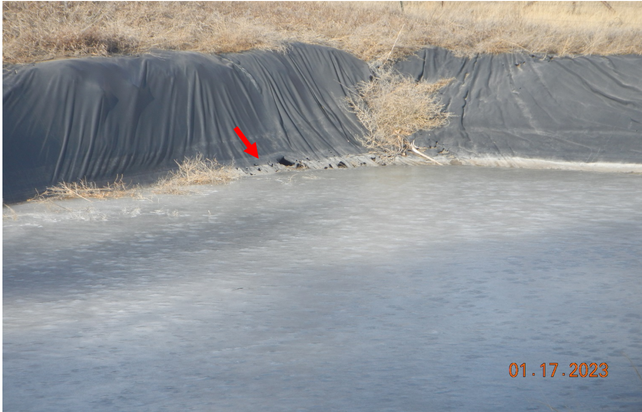
Photo 3. There are holes in the pit liner which are at the water level.
