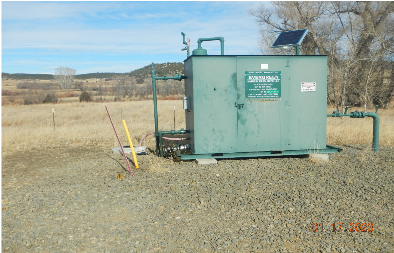
Photo 4. The well signs are posted at the meter shed. Stained soils have been cleaned up and a secondary container was installed.
