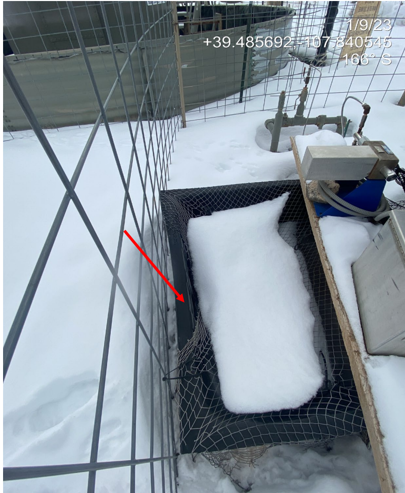
Photo 3. Photos show the wildlife protection netting is not in proper functioning condition due to being weighed down by snow.
