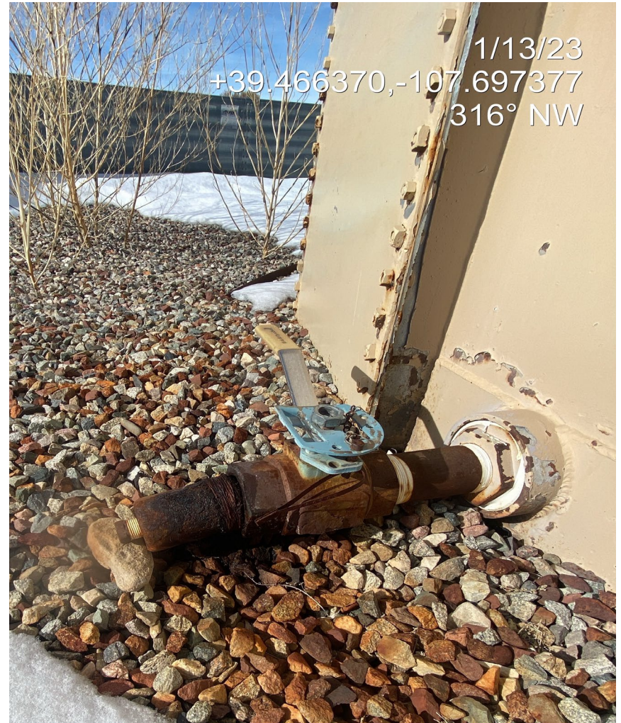
Photo 2. Photos tank battery signage is absent (left) and the tank drain line bull plug is partially ajar/not properly installed.
