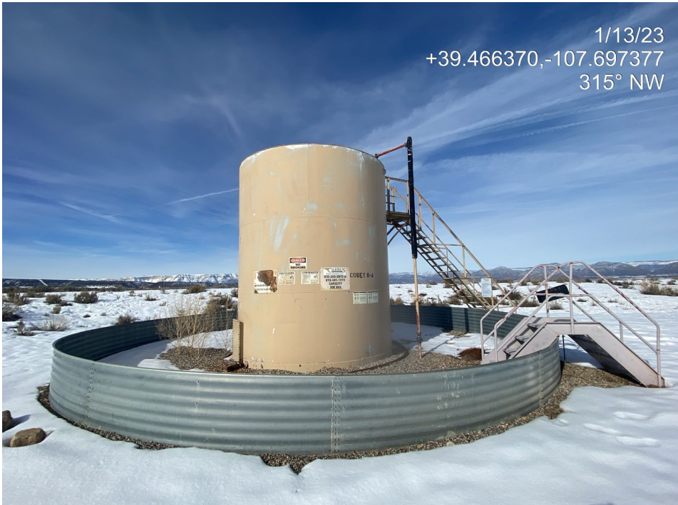
Photo 2. Photos tank battery signage is absent (left) and the tank drain line bull plug is partially ajar/not properly installed.
