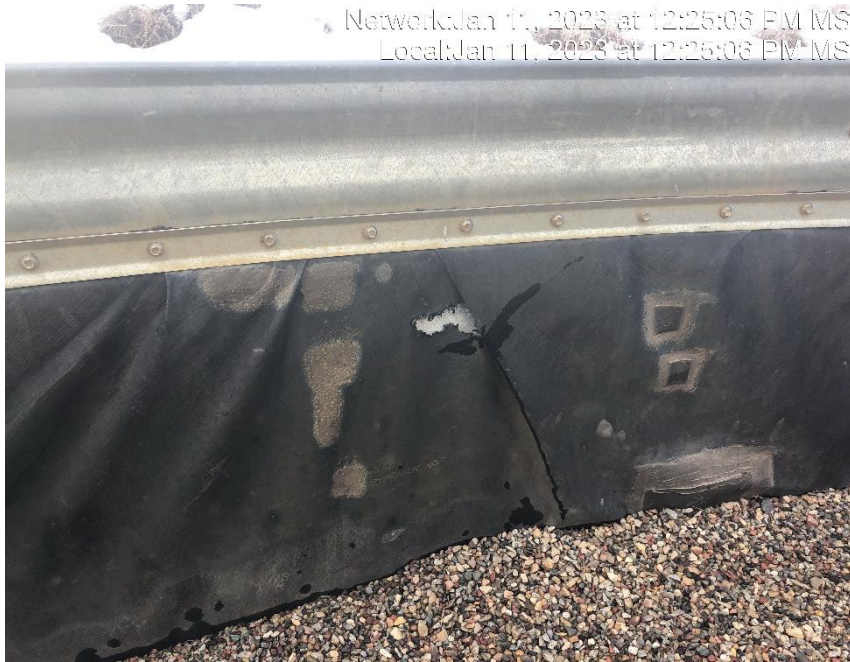
Photo #8777 Multiple holes in tank containment.
