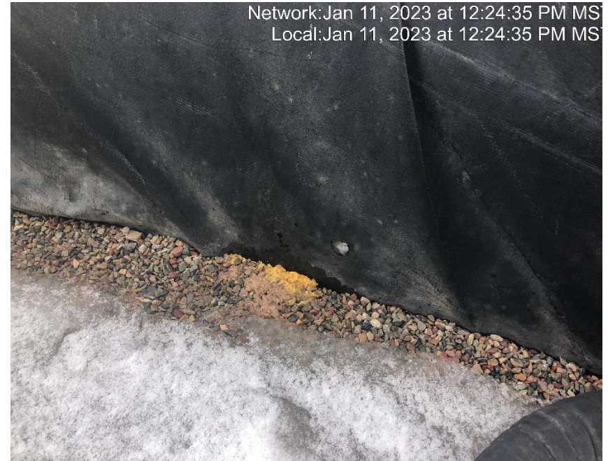
Photo #8776 Hole in secondary containment and stained gravel.
