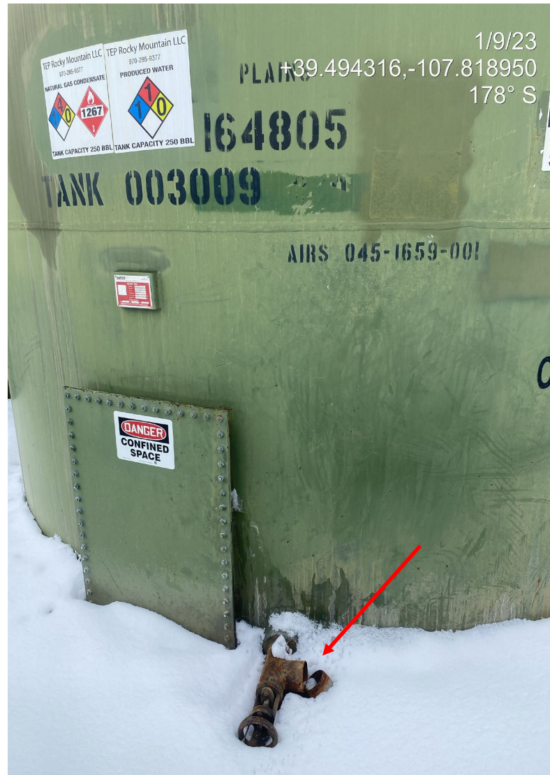
Photo 2. Photo shows a bull plug not installed.
