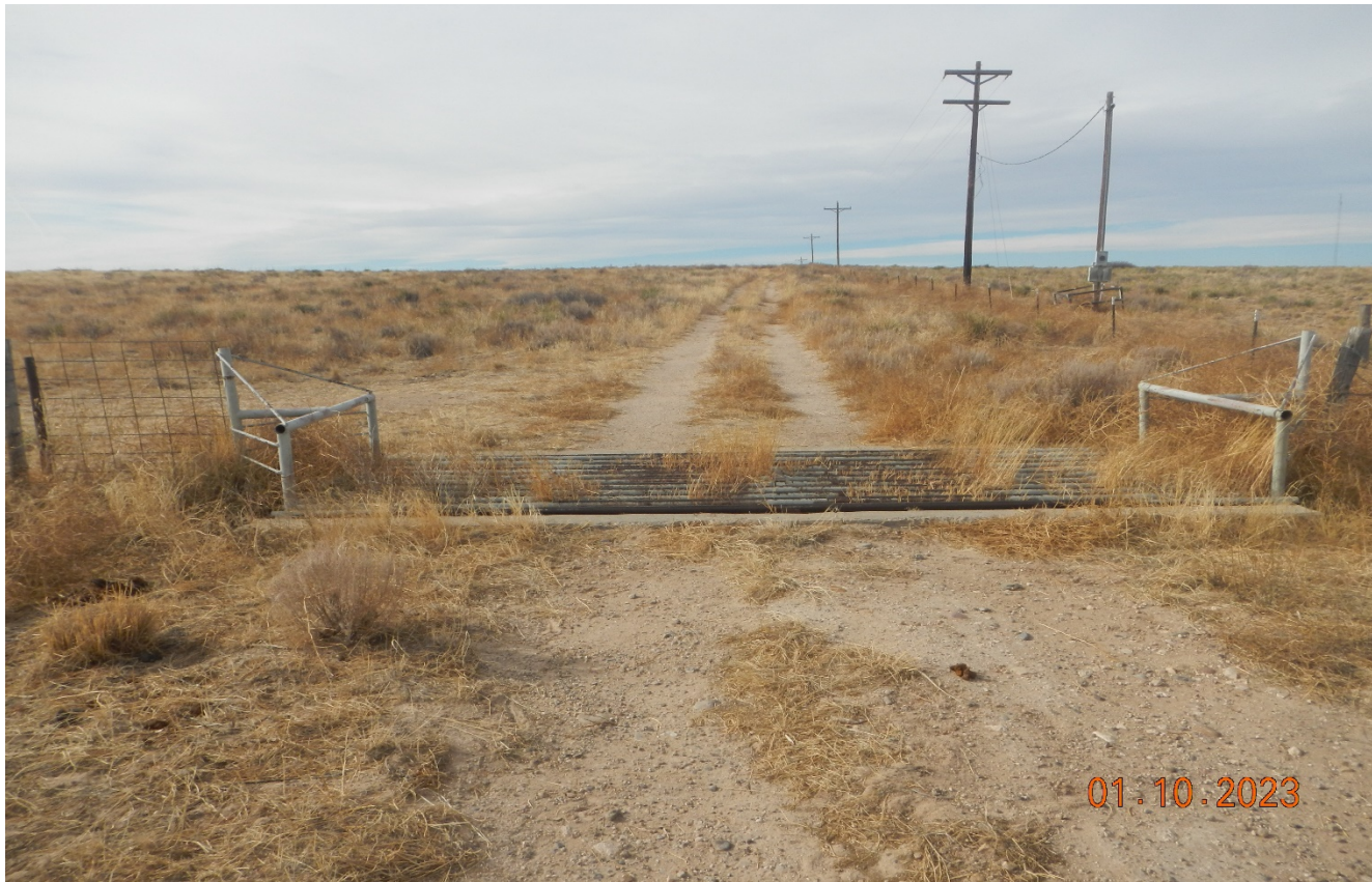
Photo 1. Facing west at the beginning of the access road. The cattle guard has not been removed and the road is not reclaimed.
