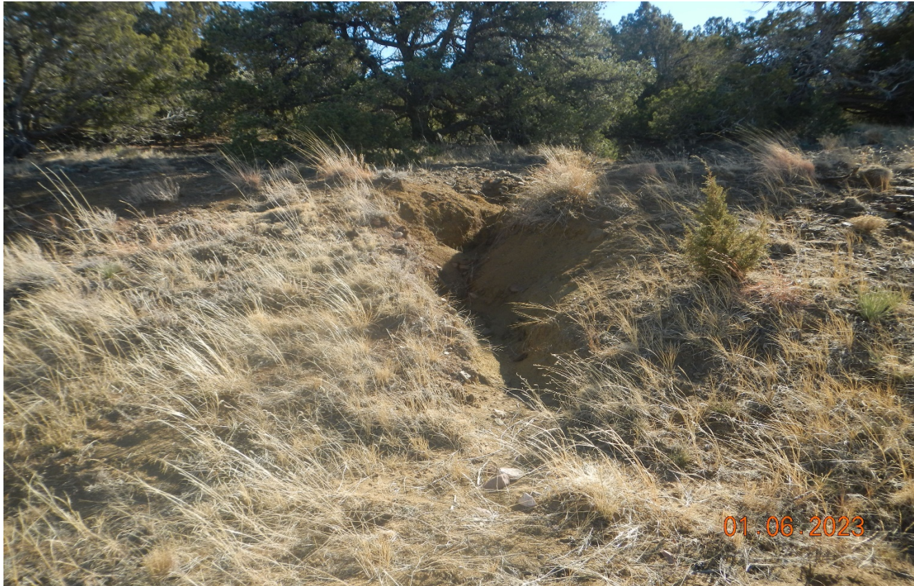
Photo 4. There is an erosion channel along the cut slope which was not repaired since previous inspection.
