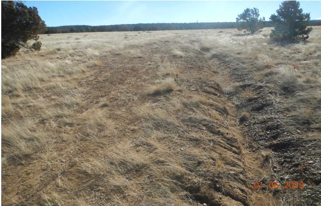
Photo 2. There is an erosion channel along the former road. This needs to be repaired and reclaimed. Previous corrective action was not completed.
