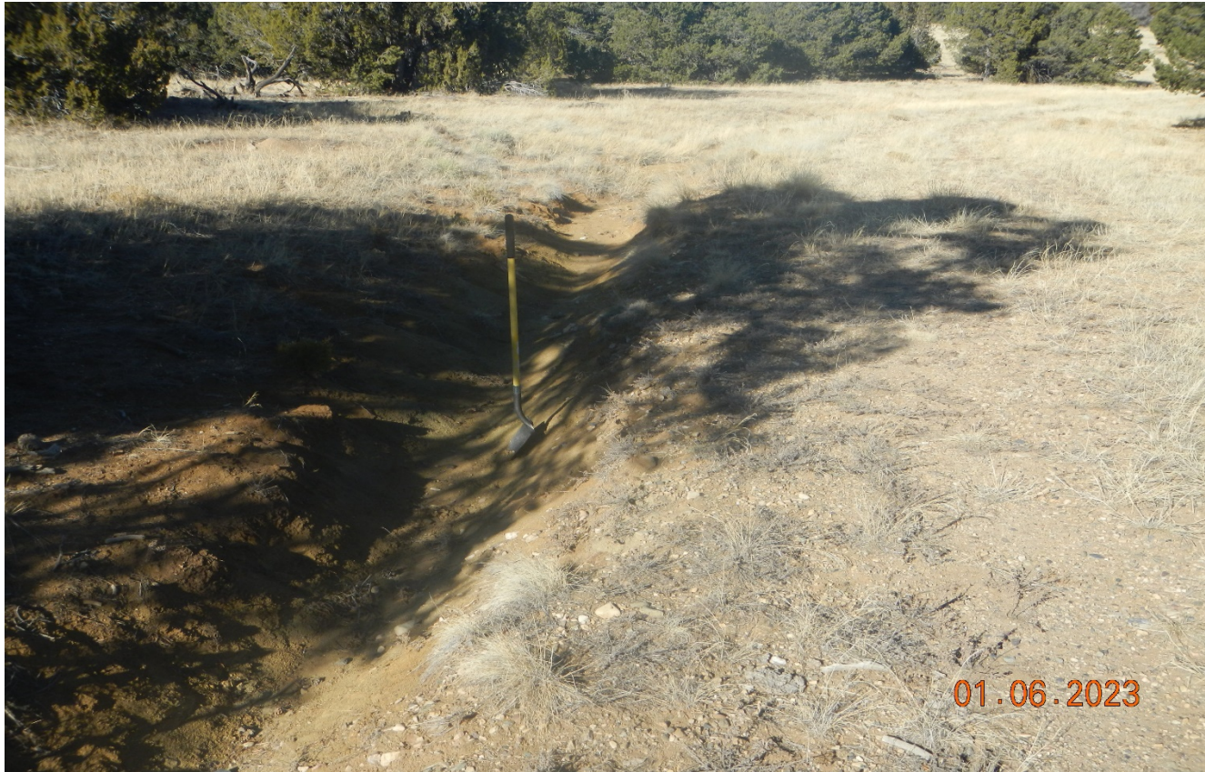
Photo 2. There is an area of erosion along the former road which has not been repaired and stabilized.
