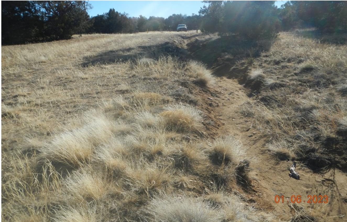
Photo 3. Facing back southeast along the road where erosion occurred along the roadside.
