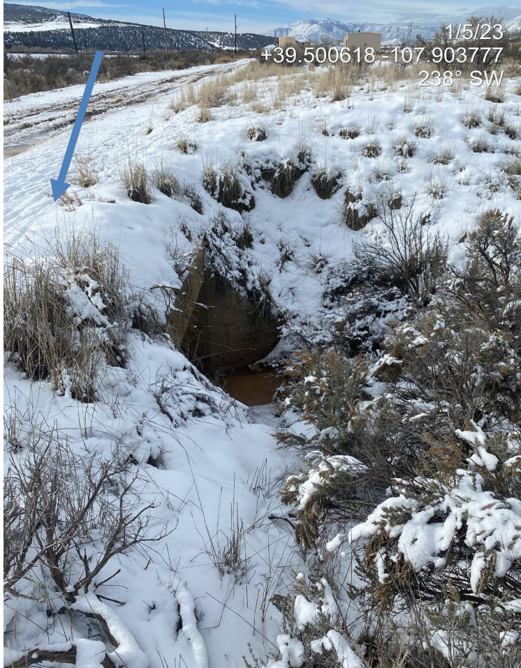
Photo 4. Photos show the access road culvert to the north (left) and south (right). No degradation observed in visible areas at the time of this inspection. Areas of previously observed rill erosion (arrow) are snow covered.
