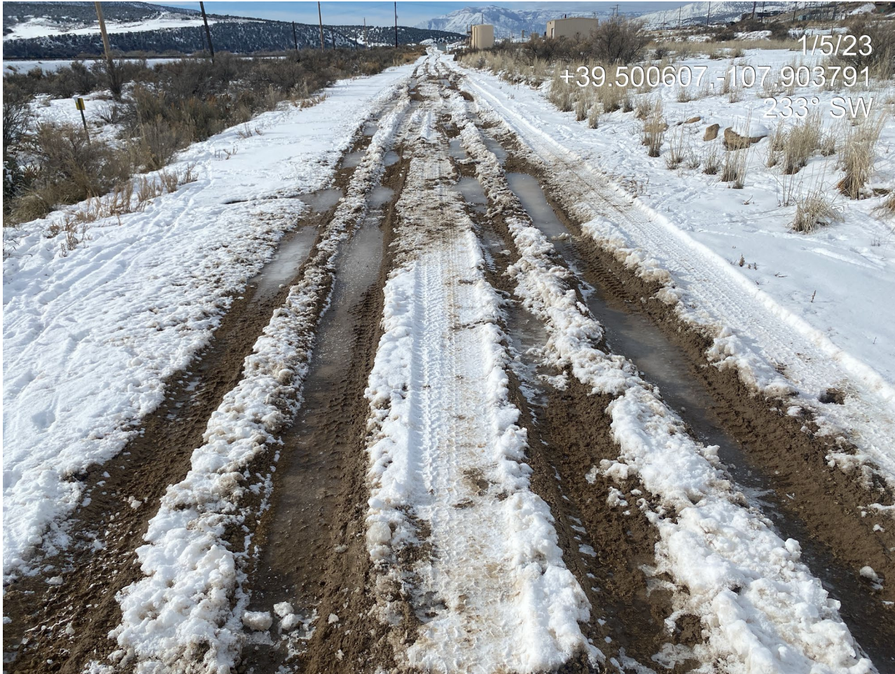
Photo 3. Photo shows degradation to the access road to the west of the location.
