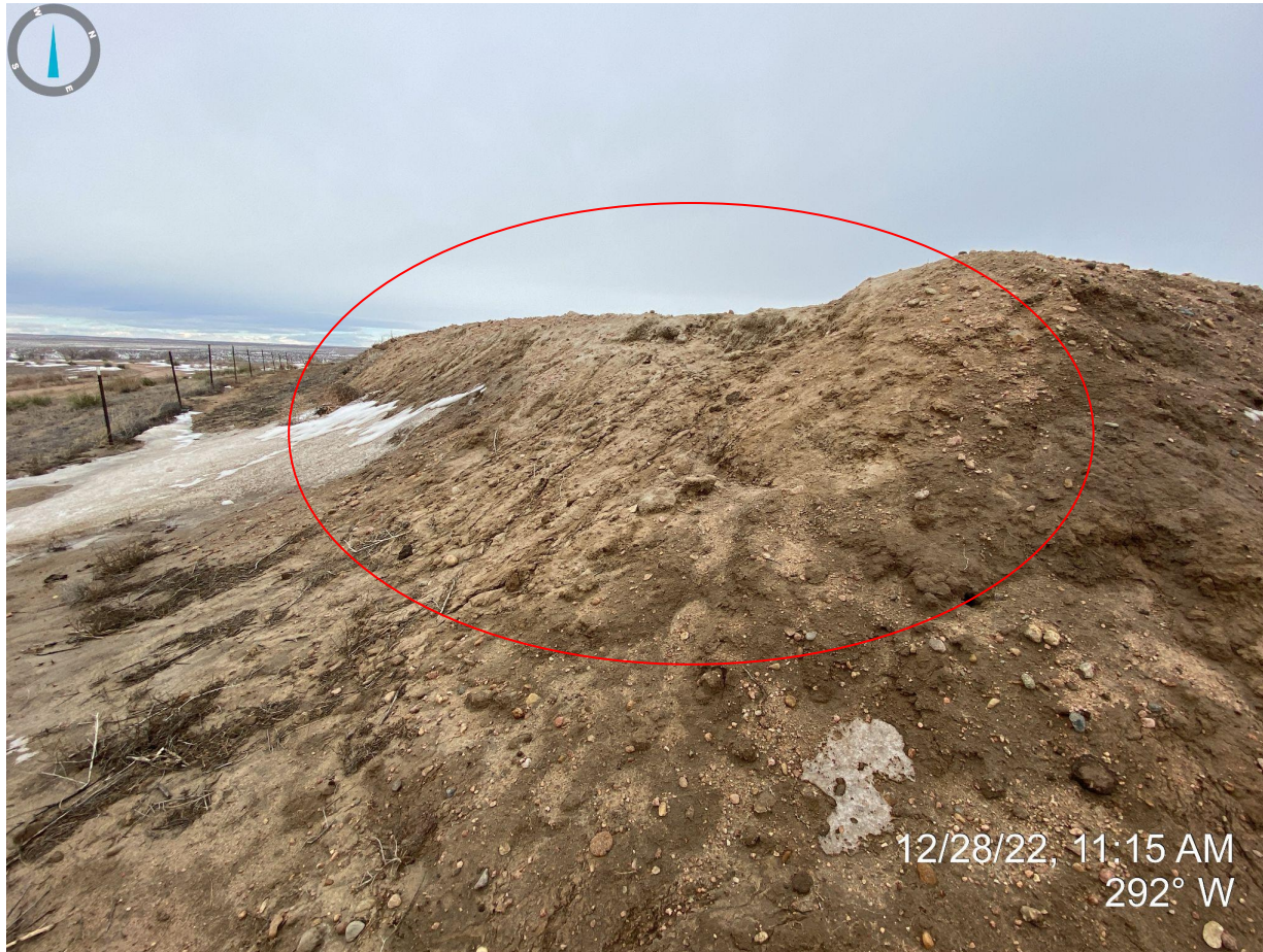
Photo 16. Facing west from the southeast corner of the pit. Photo illustrates unstabilized pit wall with evidence of rill erosion, vertical shape and unconsolidated material that is susceptible to further erosion.
