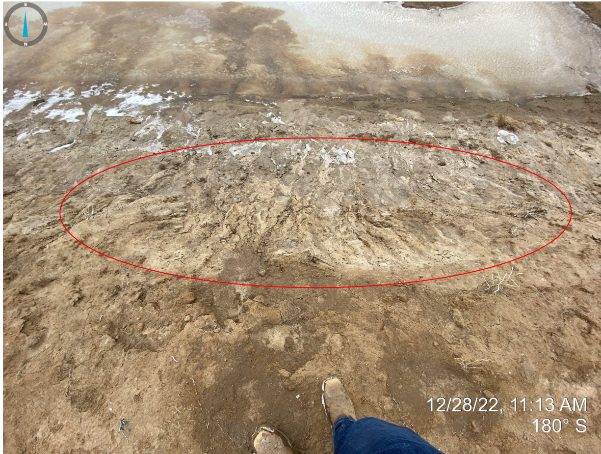
Photo 15. Facing south from northern pit wall. Photo illustrates evidence of rill erosion on the inside pit wall.
