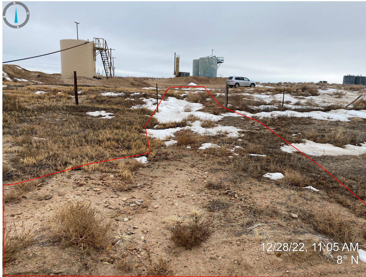
Photo 1. Facing north from access road. Photo illustrates gully erosion occurring on location and recent sediment laden stormwater migrating off location, outlined in red.
