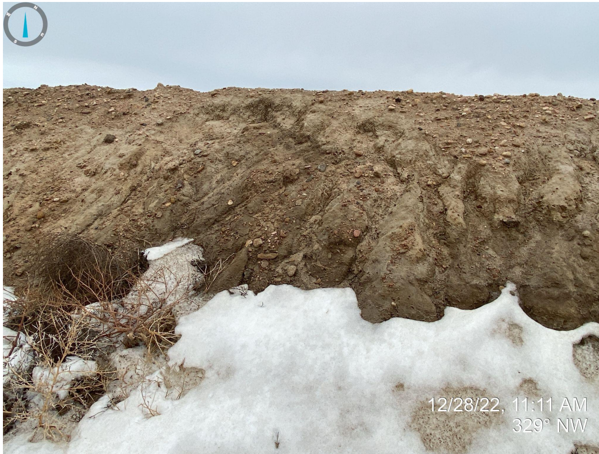
Photo 13. Facing northwest. Photo illustrates close up of unstabilized pit walls that were comprised of unconsolidated material, evidence of rill erosion, and almost vertical in shape.
