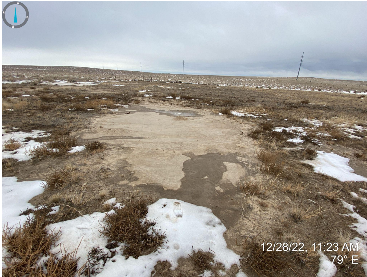
Photo 23. Facing east near the former Boxer East Skim Pit. Photo illustrates an area approximately 10' x 30' in size that is void of any vegetation, possibly a result of salt impacted soils. This area will need to be investigated and properly remediated in order to close the former skim pit (#102702).
