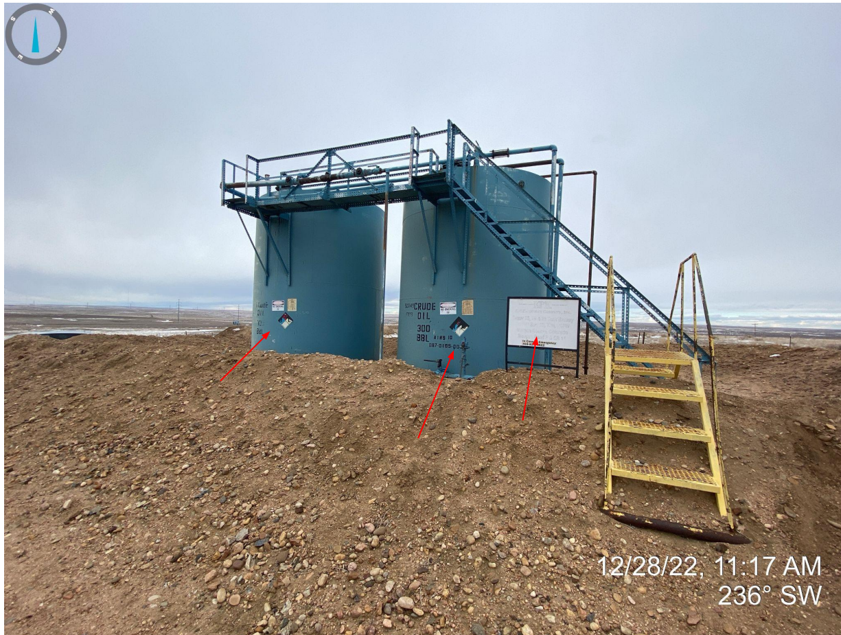
Photo 20. Facing southwest at tank battery. Photo illustrates the sign at the facility is illegible and faded, and faded/torn hazmat placards on tanks.
