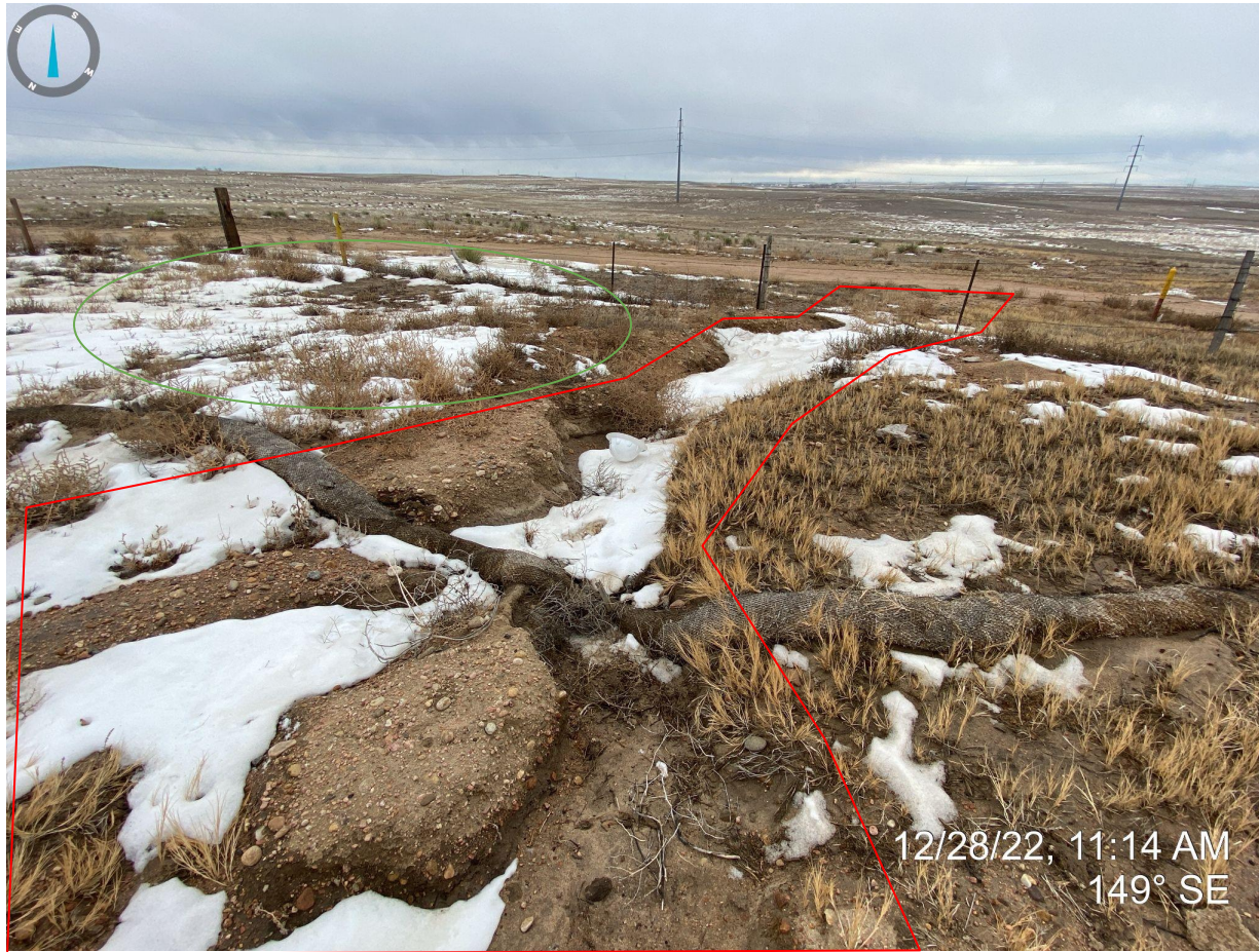
Photo 3. Facing southeast from location, near produced water pit. Photo illustrates gully erosion resulting from inadequate stormwater BMPs; e.g. degraded and improperly installed straw wattles. Also pictured, presence of russian thistle and kochia observed, outlined in green. Stormwater BMPs need to be installed and maintained in order to prevent further erosion and degradation to adjacent lands.
