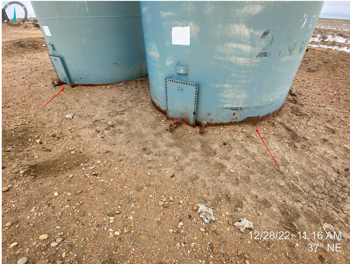
Photo 19. Facing northeast at crude tank battery facility. Photo illustrated pitted/rusted tank bottoms.
