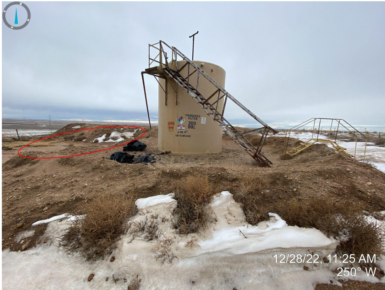
Photo 18. Facing west towards produced water tank. Photo illustrates no emergency contact information posted at facility, evidence of undesirable vegetation (e.g. russian thistle and kochia), debris (plastic liner), and a breached earthen berm with inadequate free board.
