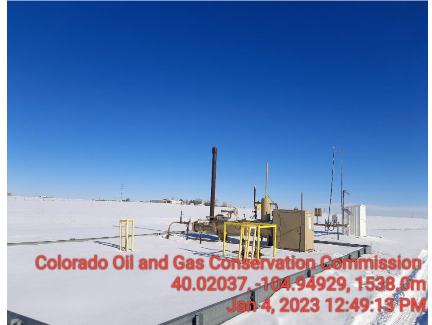
Photo 4 production equipment and meter house.
