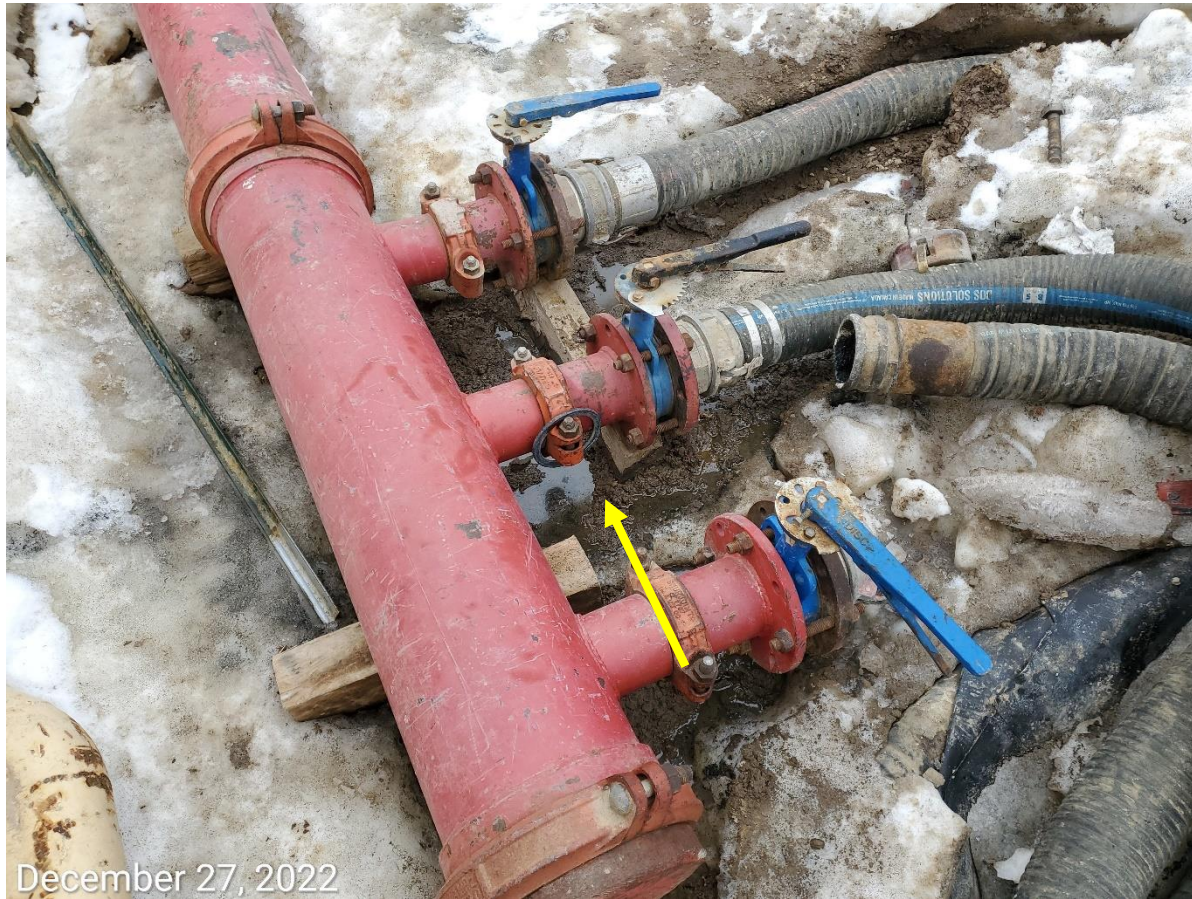
Photo 4: Photo shows connection points at pipes adjacent to the produced water tanks on the southwest end of the Location. Fluids were observed releasing onto the pad surface.
