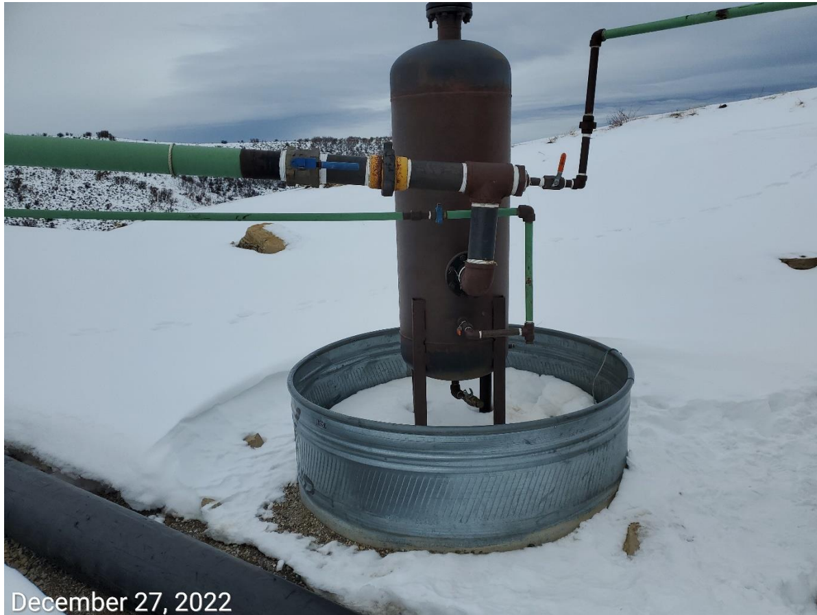
Photo 8: Photo shows wildlife protection devices missing from containment BMP.
