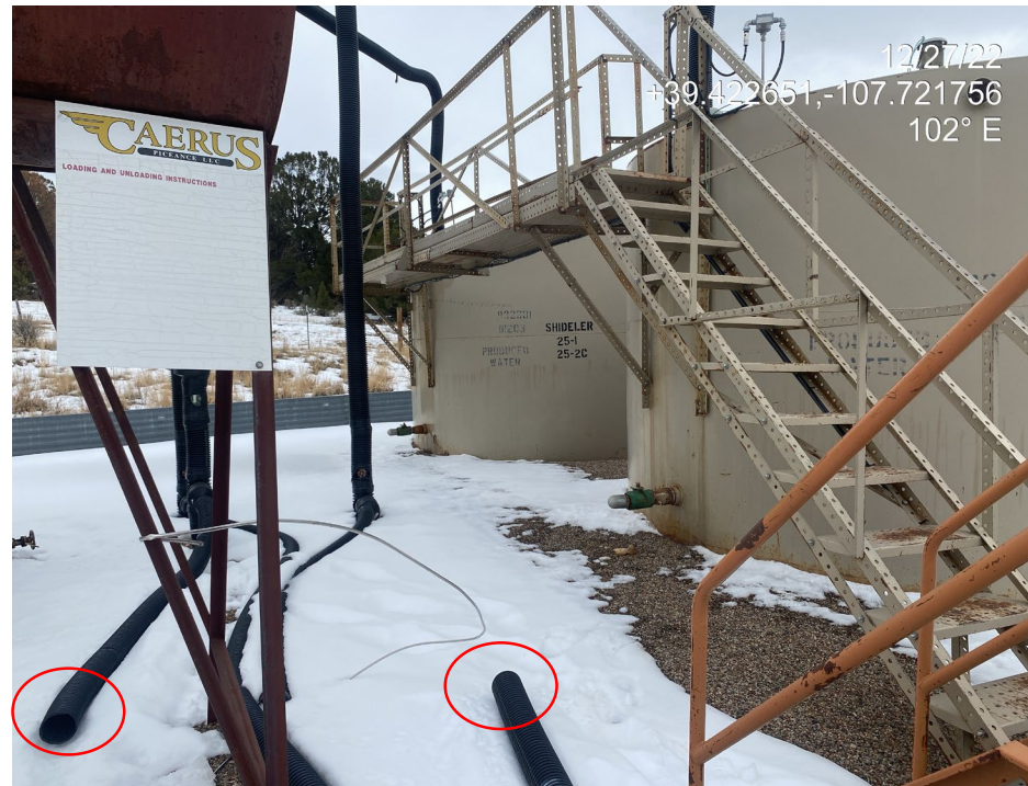
Photo 2. Photos show bull plugs not installed on tank drain lines (left) and open ended piping at tank battery (right).
