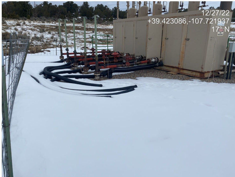
Photo 3. Photos shows open ended piping at separators.
