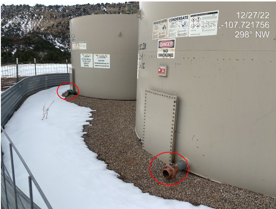
Photo 2. Photos show bull plugs not installed on tank drain lines (left) and open ended piping at tank battery (right).
