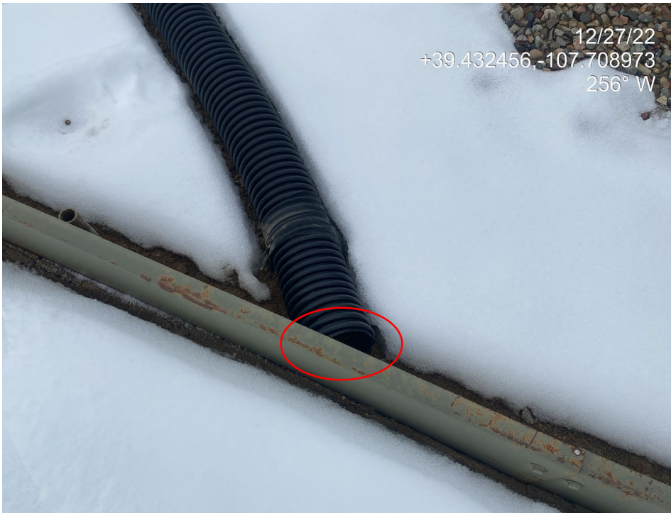
Photo 3. Photos show open ended separator piping.
