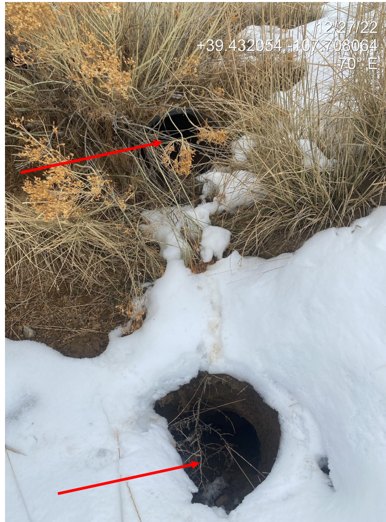
Photo 4. Photo shows a plastic drain pipe (top) being bypassed by stormwater resulting in undermining and erosion beneath the pipe (bottom).
