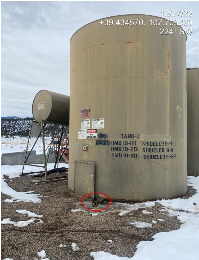
Photo 3. Photos show open ended piping and bull plugs not installed at tanks.
