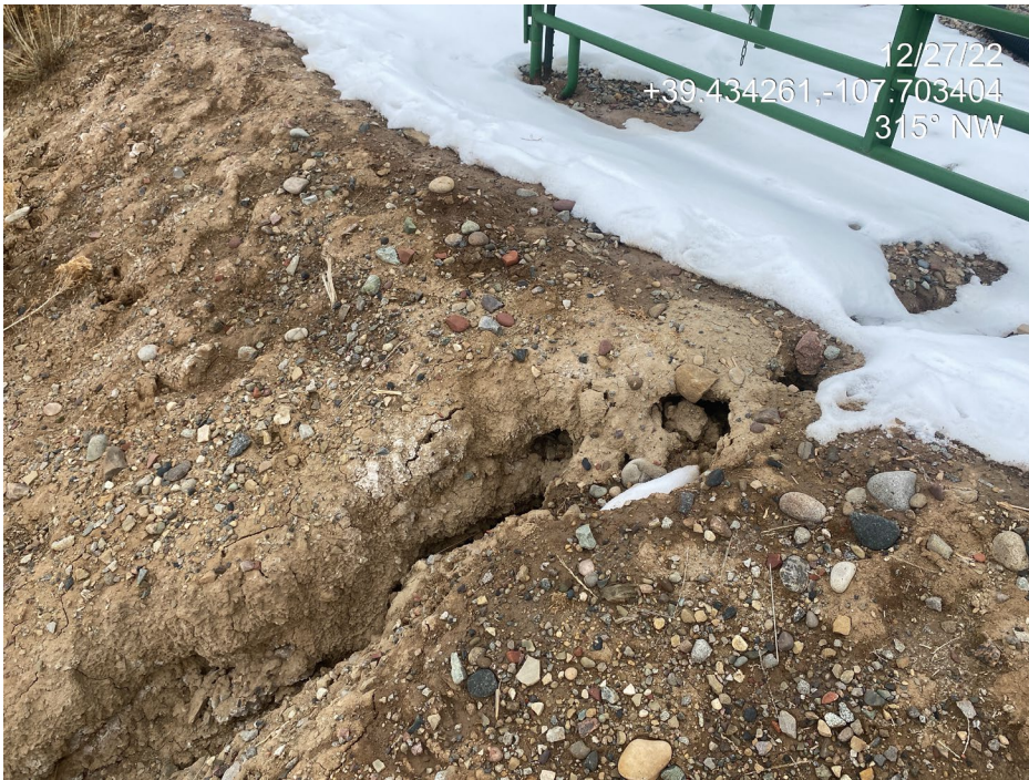
Photo 4. Photos show rill erosion behind the separators.
