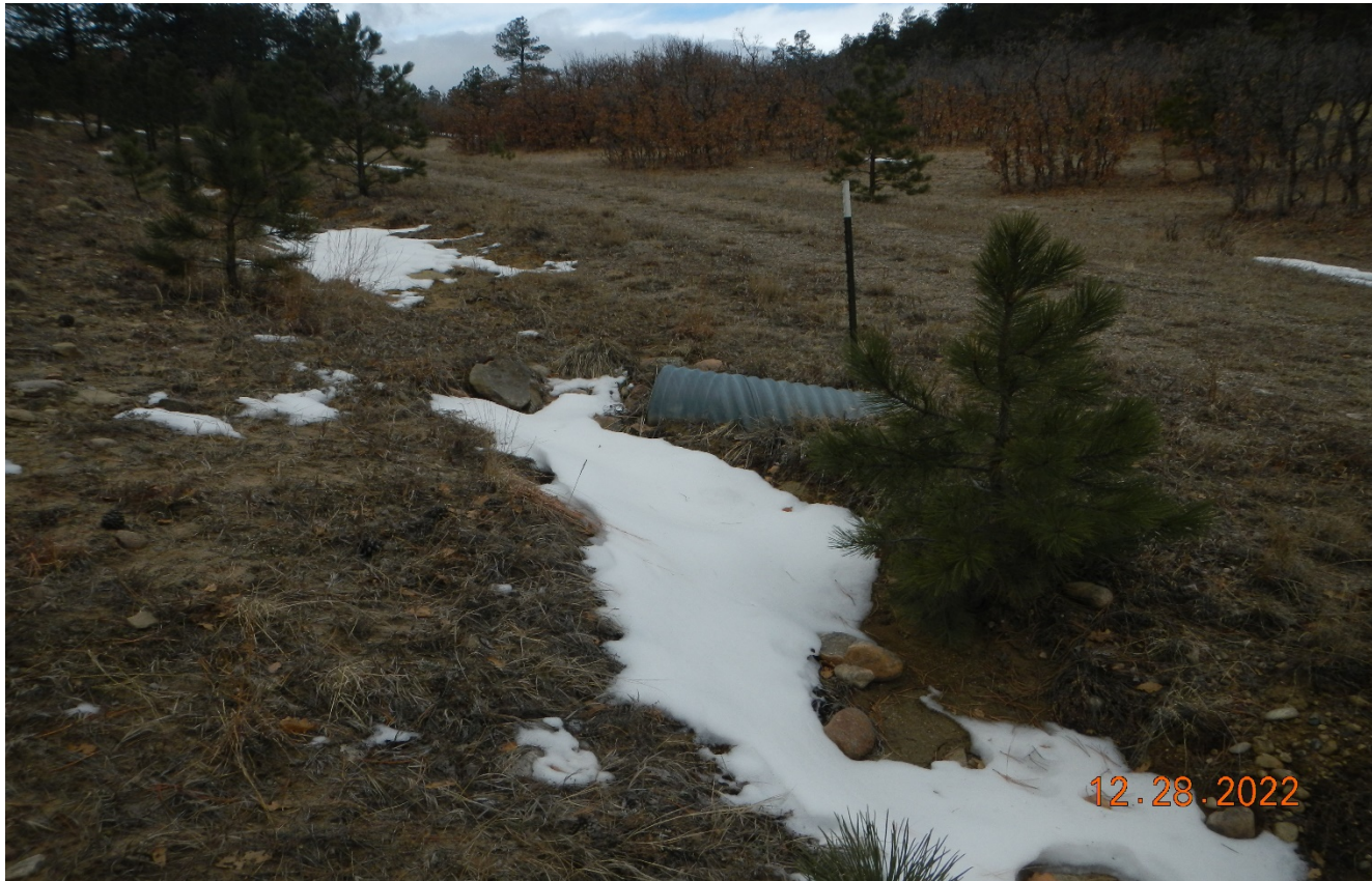
Photo 3. Further up the road is a culvert where stormwater is bypassing. This needs to be dug out to allow stormwater flow.
