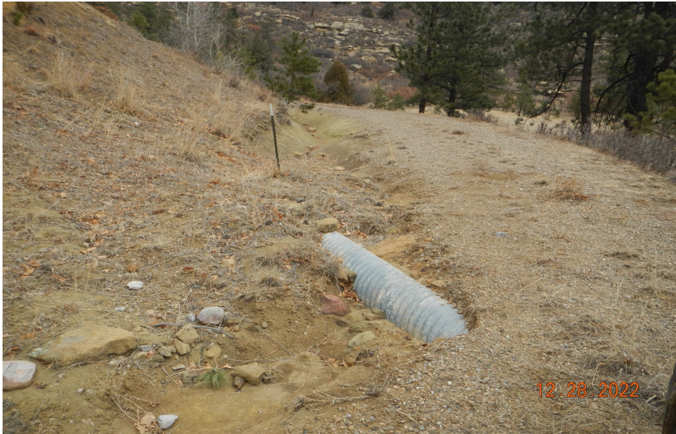
Photo 2. There is erosion along the road side that needs to be repaired and stabilized. Previous corrective action was not completed.
