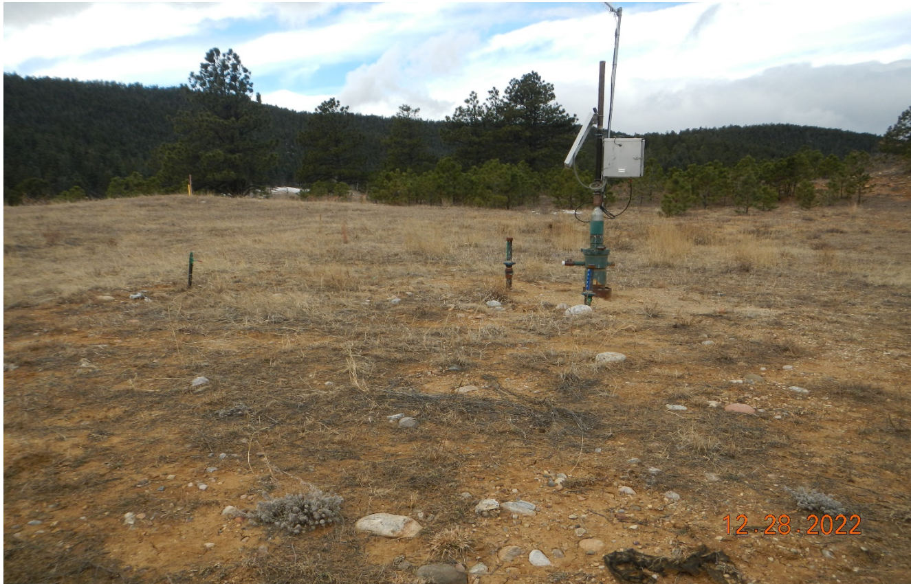
Photo 5. Facing toward the well. The 3 risers have been capped and labeled.
