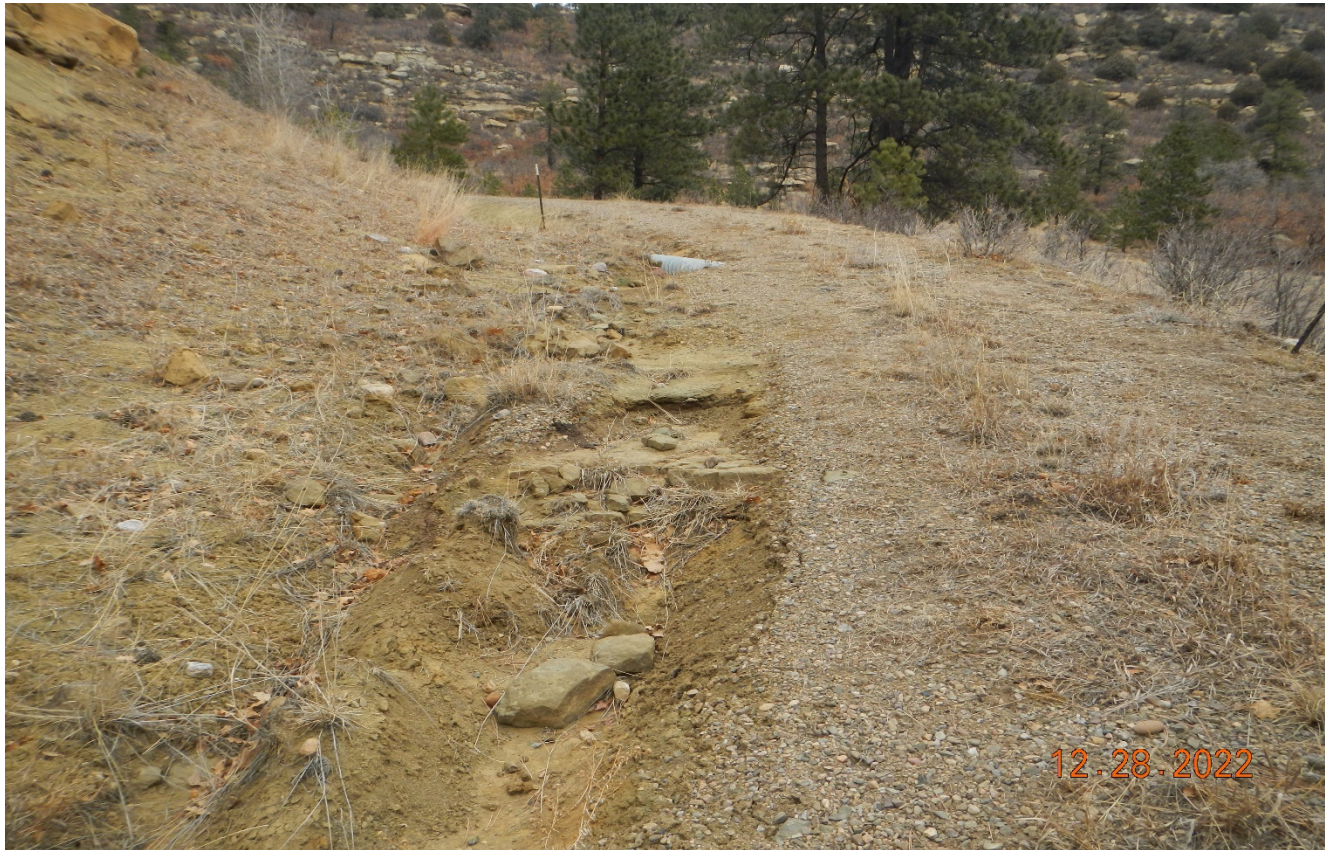
Photo 1. Facing north along the access road. Stormwater is bypassing the culvert causing erosion down the road. Previous corrective action was not completed.
