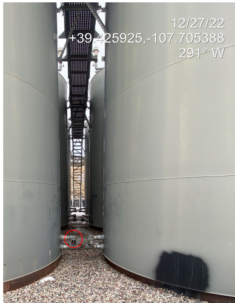
Photo 4. Photos show bull plugs not installed on tank drain line.
