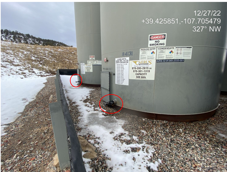
Photo 4. Photos show bull plugs not installed on tank drain line.
