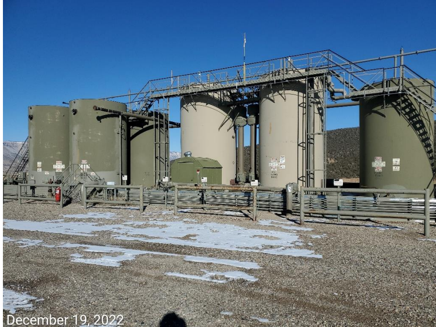
Photo 5: Northeastern tank battery facility. Photo right shows tanks missing signage/labeling.
