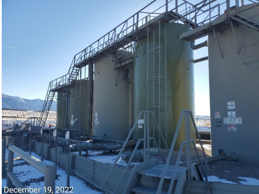
Photo 4: Western Tank battery Facility. Photo right shows southern-most tank missing signage/labeling.
