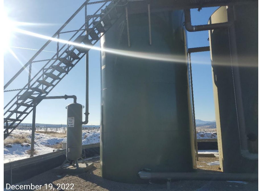
Photo 4: Western Tank battery Facility. Photo right shows southern-most tank missing signage/labeling.
