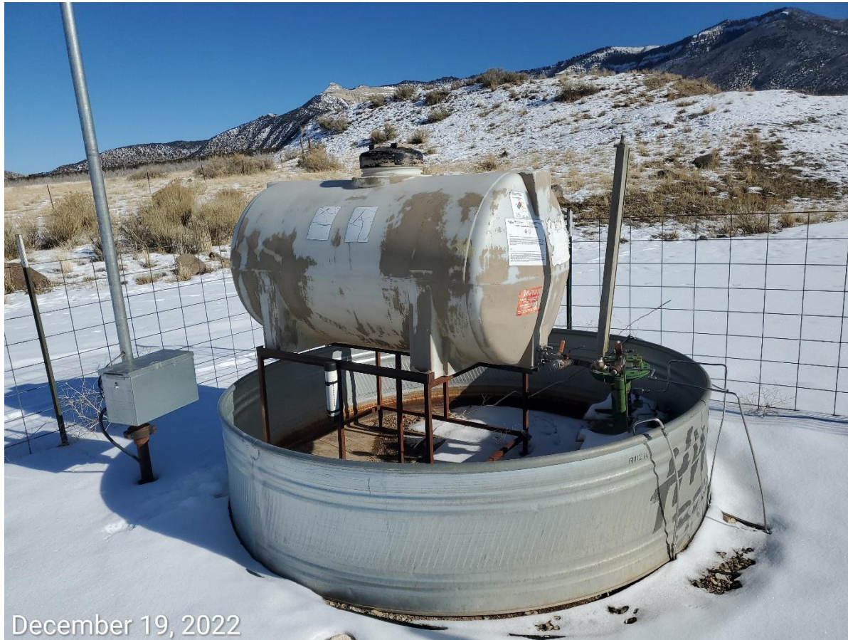
Photo 6: H2S Scavenger tank. Wildlife protection devices to prevent wildlife access to the secondary containment of the "H2S Scavenger" tank missing or insufficient.
