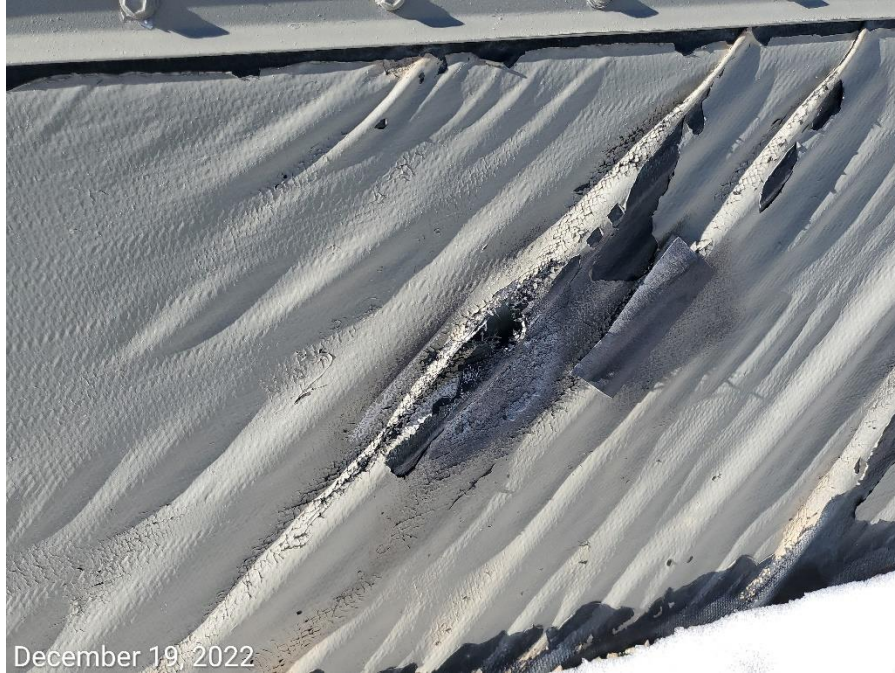
Photo 5: Photo example showing holes observed throughout entire liner at the tank battery.
