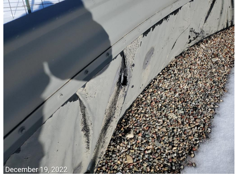
Photo 5: Photo example showing holes observed throughout entire liner at the tank battery.
