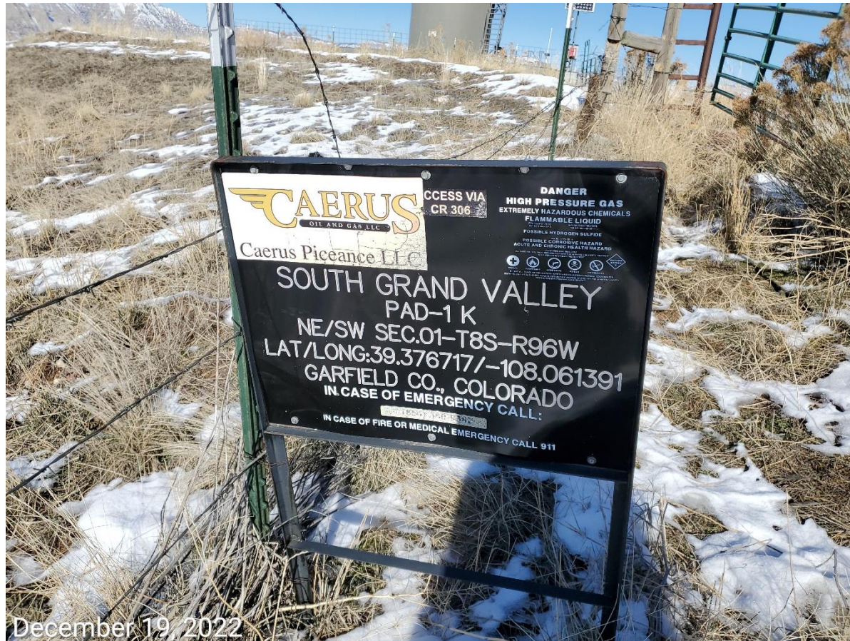
Photo 3: Signage at Location entrance. Emergency contact number no longer legible. Battery signage indicates presence of H 2 S; H 2 S signage at Location entrance not posted.
