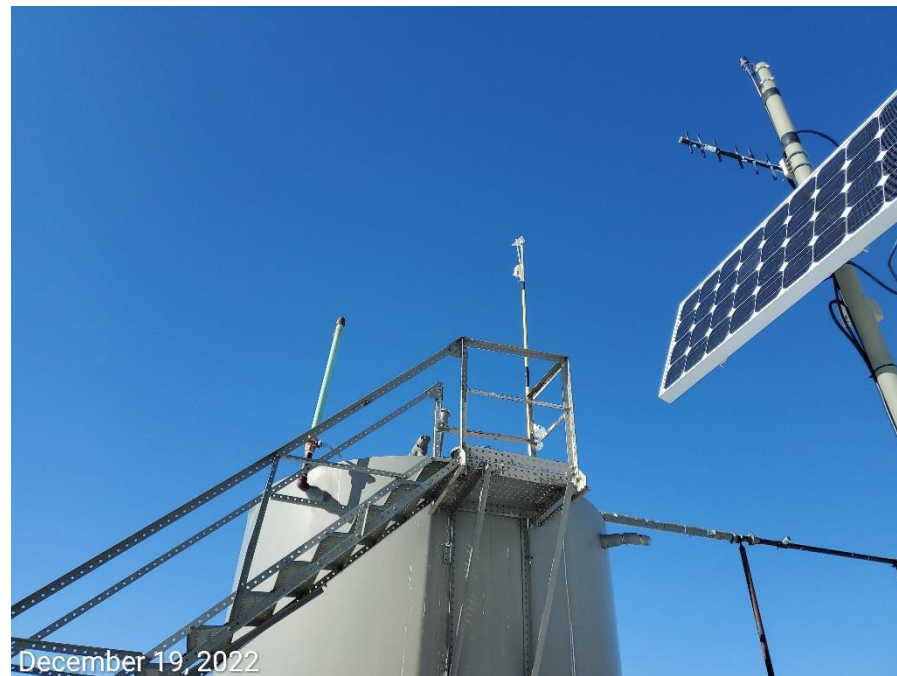
Photo 4: Tank battery. Signage at battery indicates presence of H2S. Photo right shows Wind Direction Indicator on Location is not longer in proper functioning condition.
