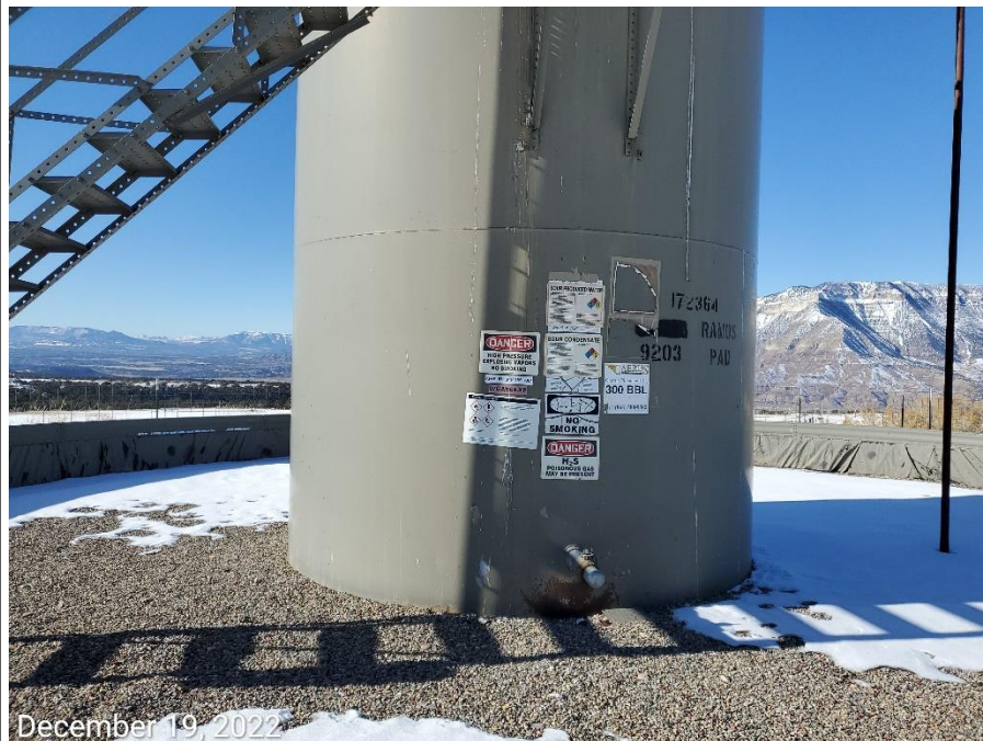
Photo 4: Tank battery. Signage at battery indicates presence of H2S. Photo right shows Wind Direction Indicator on Location is not longer in proper functioning condition.
