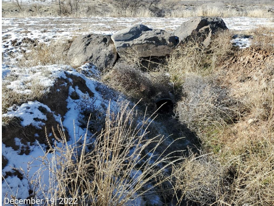
Photo 7: Weed debris accumulation at culvert.
