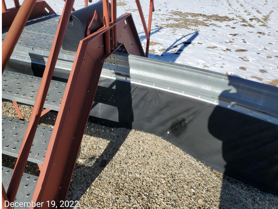
Photo 3: Photos examples showing various holes observed throughout the entire liner at the tank battery.
