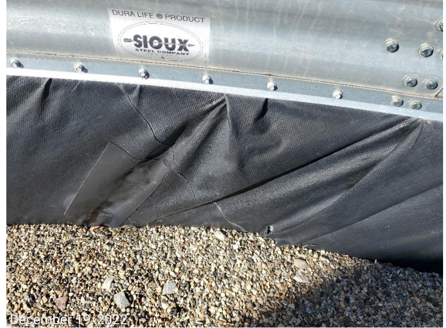
Photo 3: Photos examples showing various holes observed throughout the entire liner at the tank battery.
