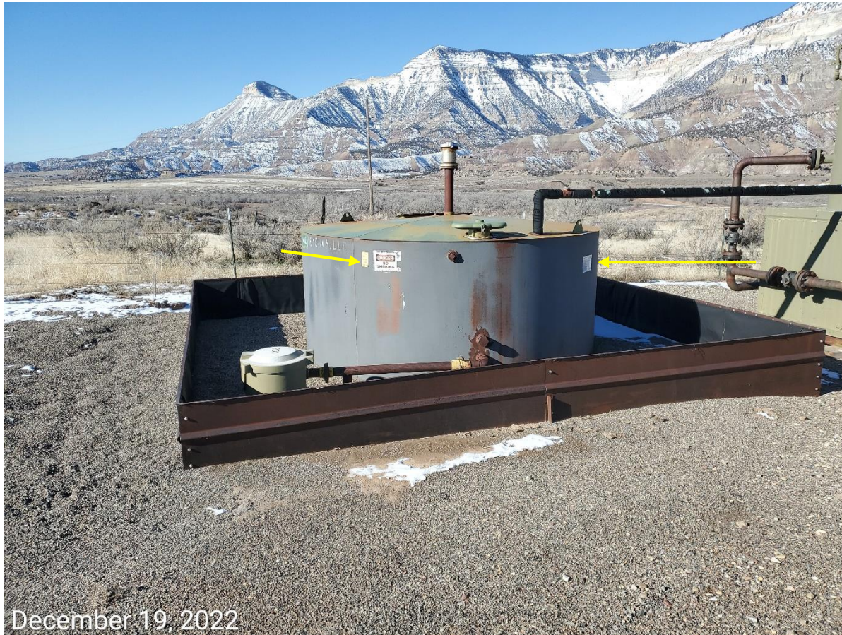
Photo 4: Laramie tank on the north end of the Location. Operator/Contents label not legible from distance (yellow arrow). Capacity label not observed.
