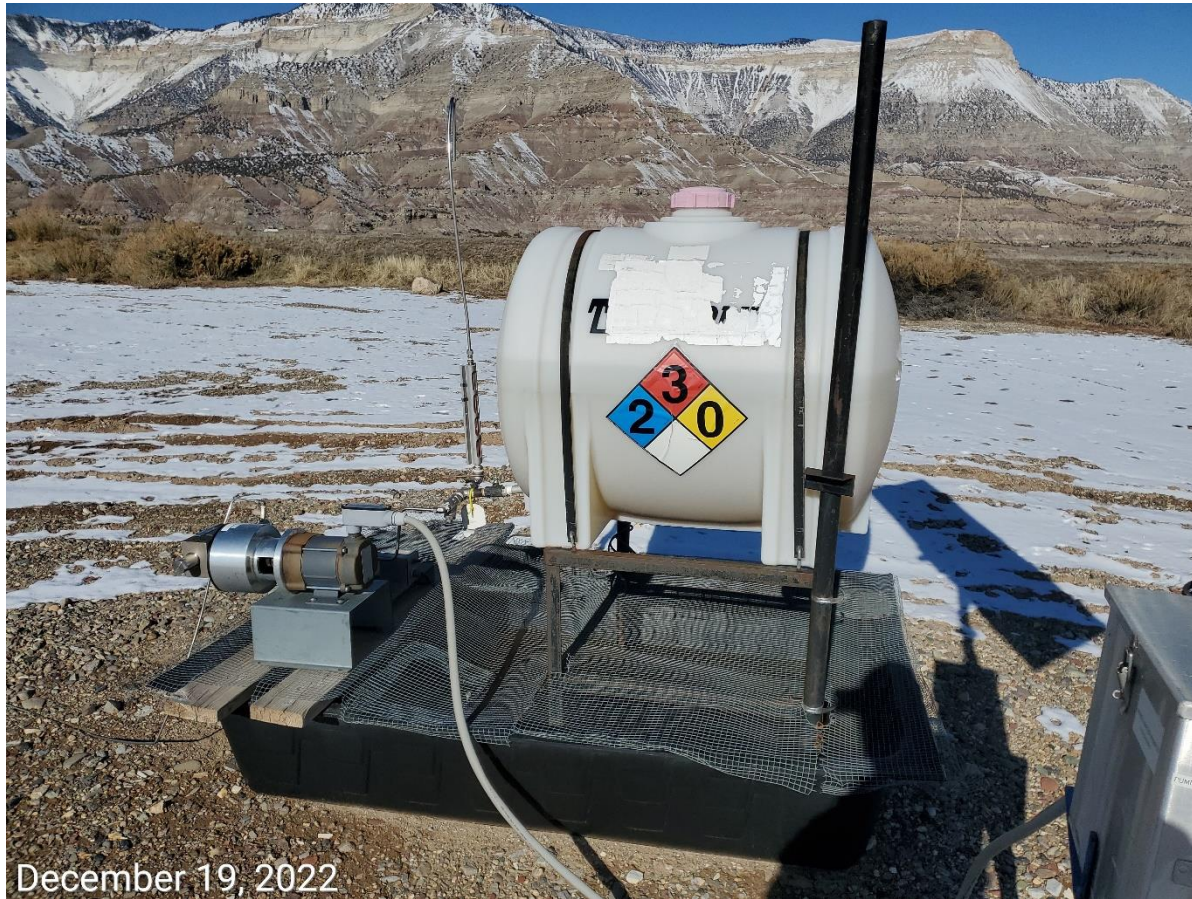
Photo 5: Tank next to wellhead. Labeling no longer legible.
