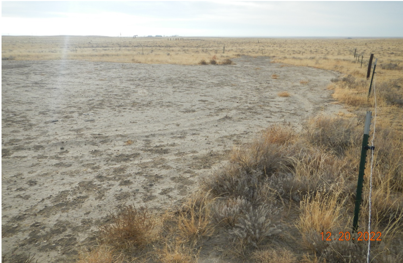
Photo 4. Facing south at the recontoured battery site. There are no stormwater controls installed down gradient and bare soils are susceptible to erosion.
