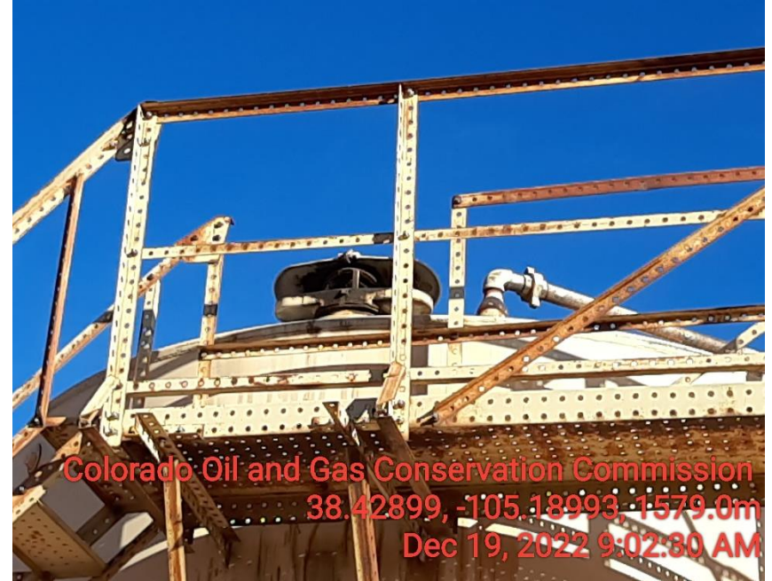
Photo 2 Gauge hatch open
