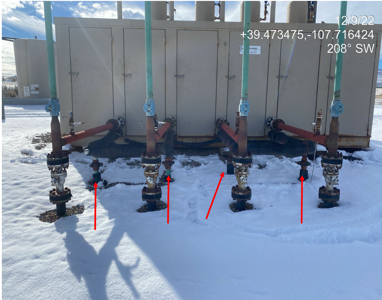
Photo 2. Photos show what appears to be four (4) unused risers.
