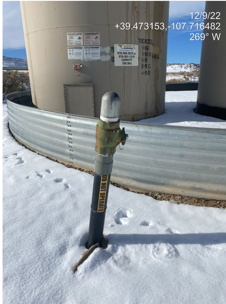
Photo 1. Photo shows a LOTO riser adjacent to the tank battery. Unused riser equipment must be removed.
